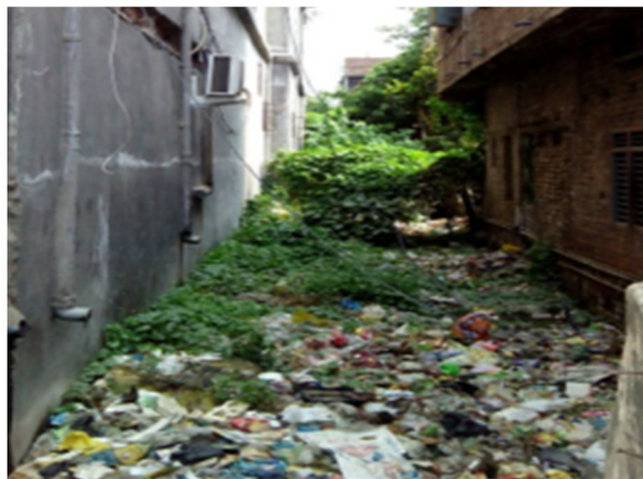
Figure 25 Choked drain Garibsthan area (Muzaffarpur)
