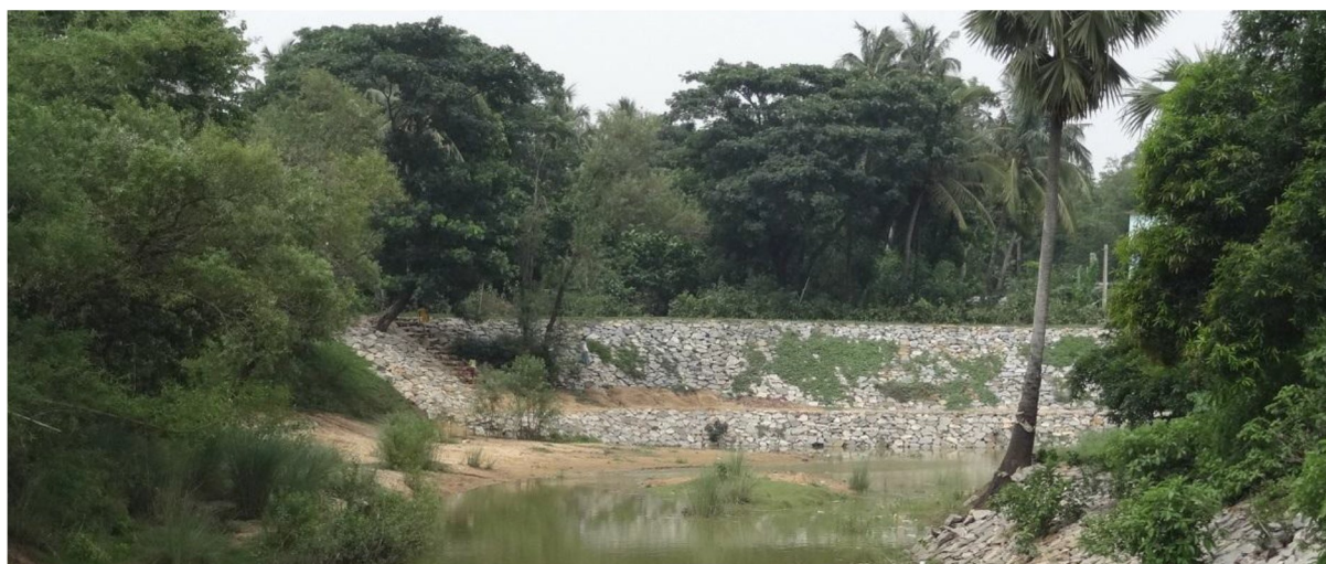
Figure 23 Embankment with revetments in stone (Jajpur district, Odisha)
