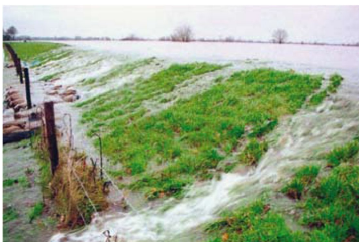
Figure 21 Overtopping of an embankment (Source: Deltares)
