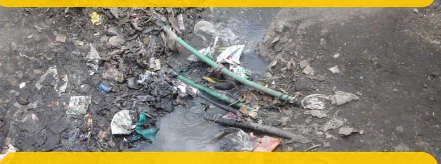
...failures of these pipes would draw waste water into the drinking water supply
