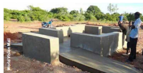
Figure 3 Ramped access to a tapstand in Mali (Source: WaterAid)
