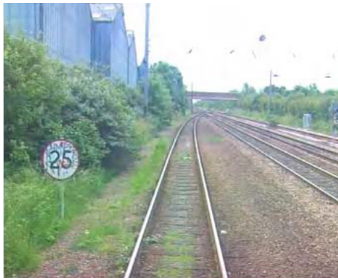
Figure 11: Full-size permissible speed indicator at Fletton Junction in 2002 (image courtesy of Network Rail)
