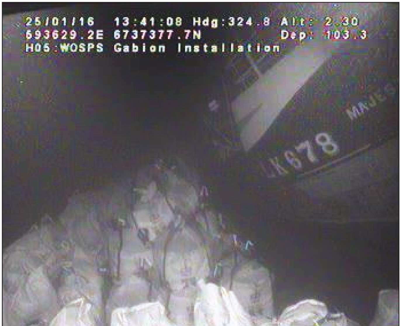
Figure 5: Sandbags positioned against the wreck
