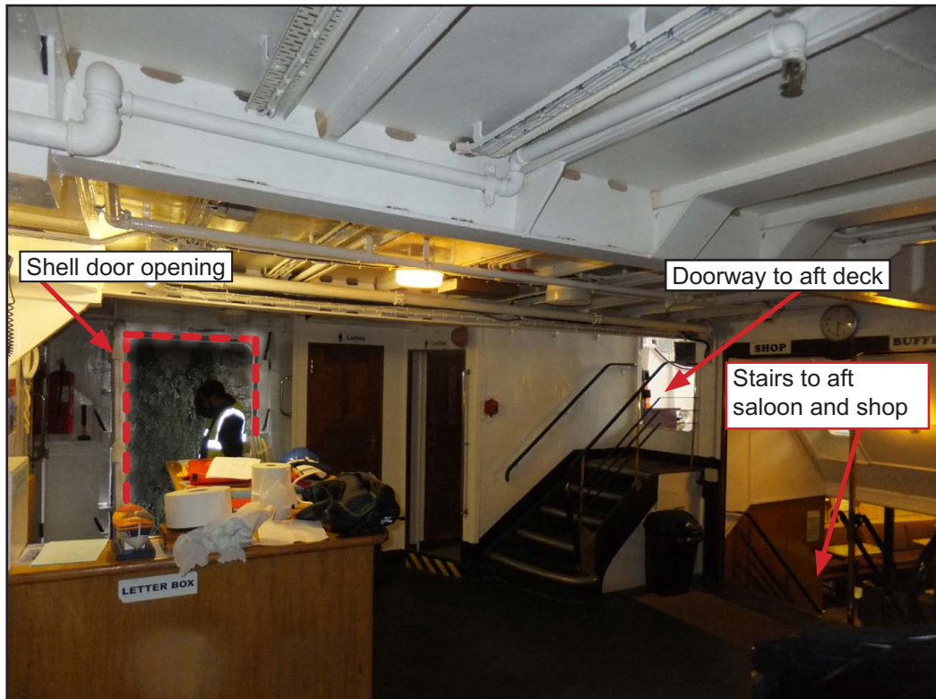
Figure 4: Starboard shell door opening, from saloon area
