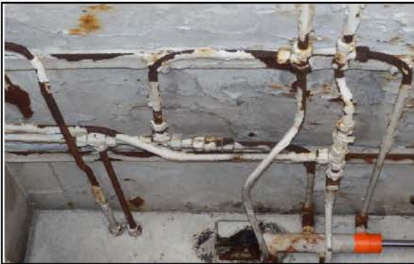
Ref. 4.2 Example of hyd. Pipe condition
