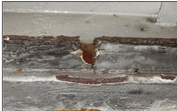
Ref. 3.5 Guide rail piece missing
