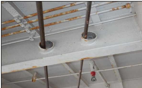
Ref. 3.1 No protection on wire ropes
