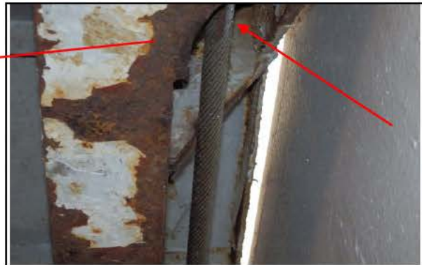
Ref. 3.9 Wire fouling under tension
