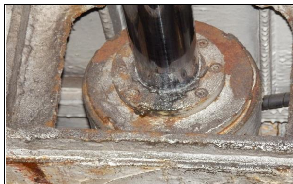
Ref. 3.4 Gland seal leaking
