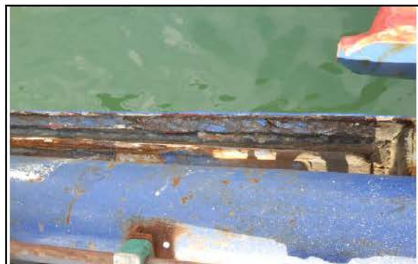
Ref. 1.4 Seal cracked and painted
