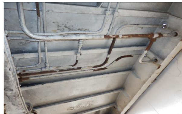
Ref. 3.3 Example of corroding pipe runs
