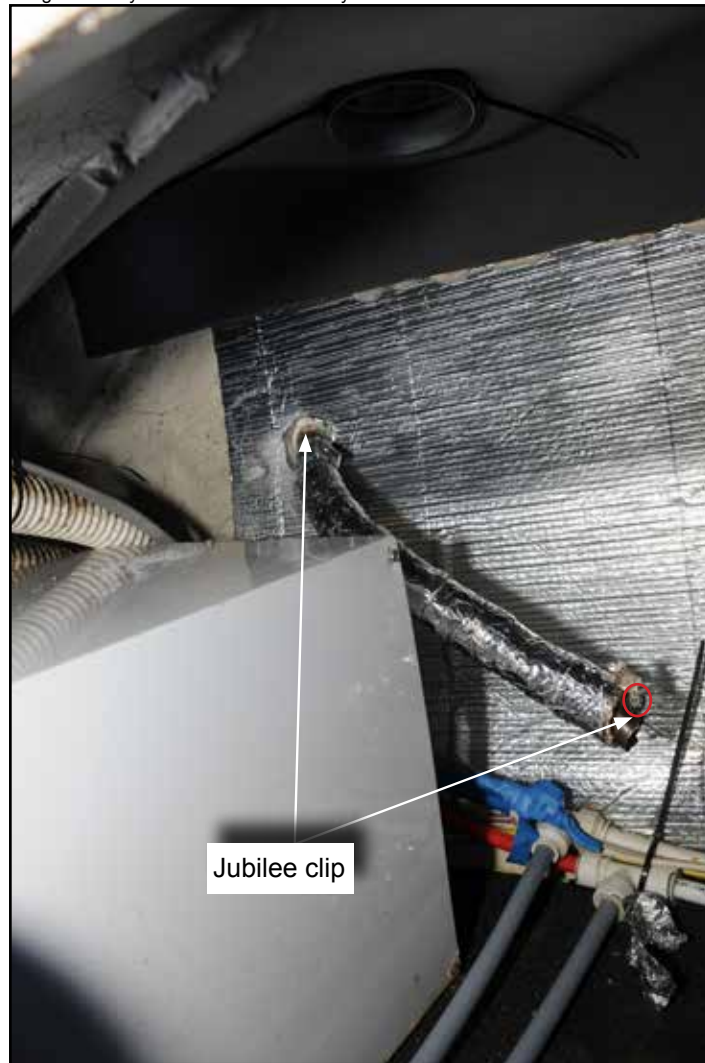
Figure 11: Silencer to through hull fitting
