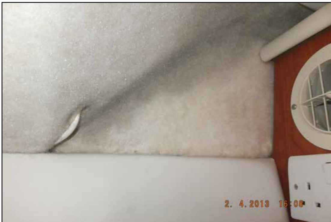
Figure 23: Deckhead lining - gas staining
