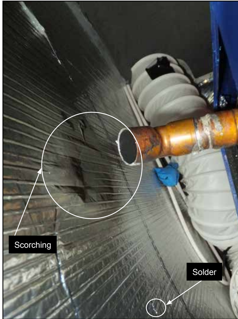
Figure 17: Solder splash on engine bay bulkhead
