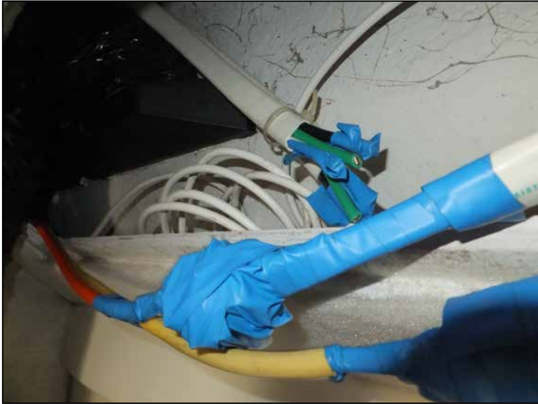
Figure 13: Electrical wire joints
