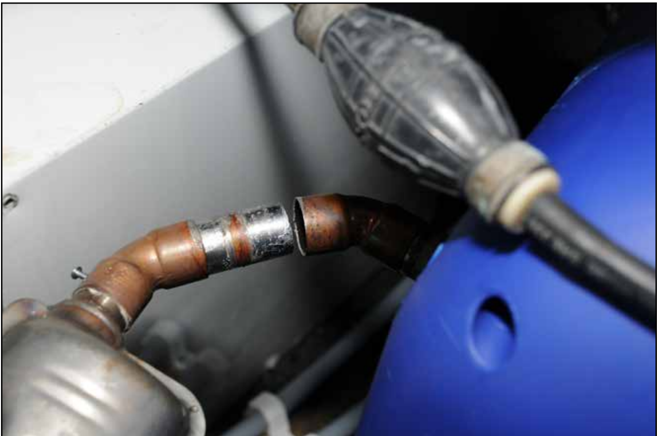
Figure 10: Failed soldered joint
