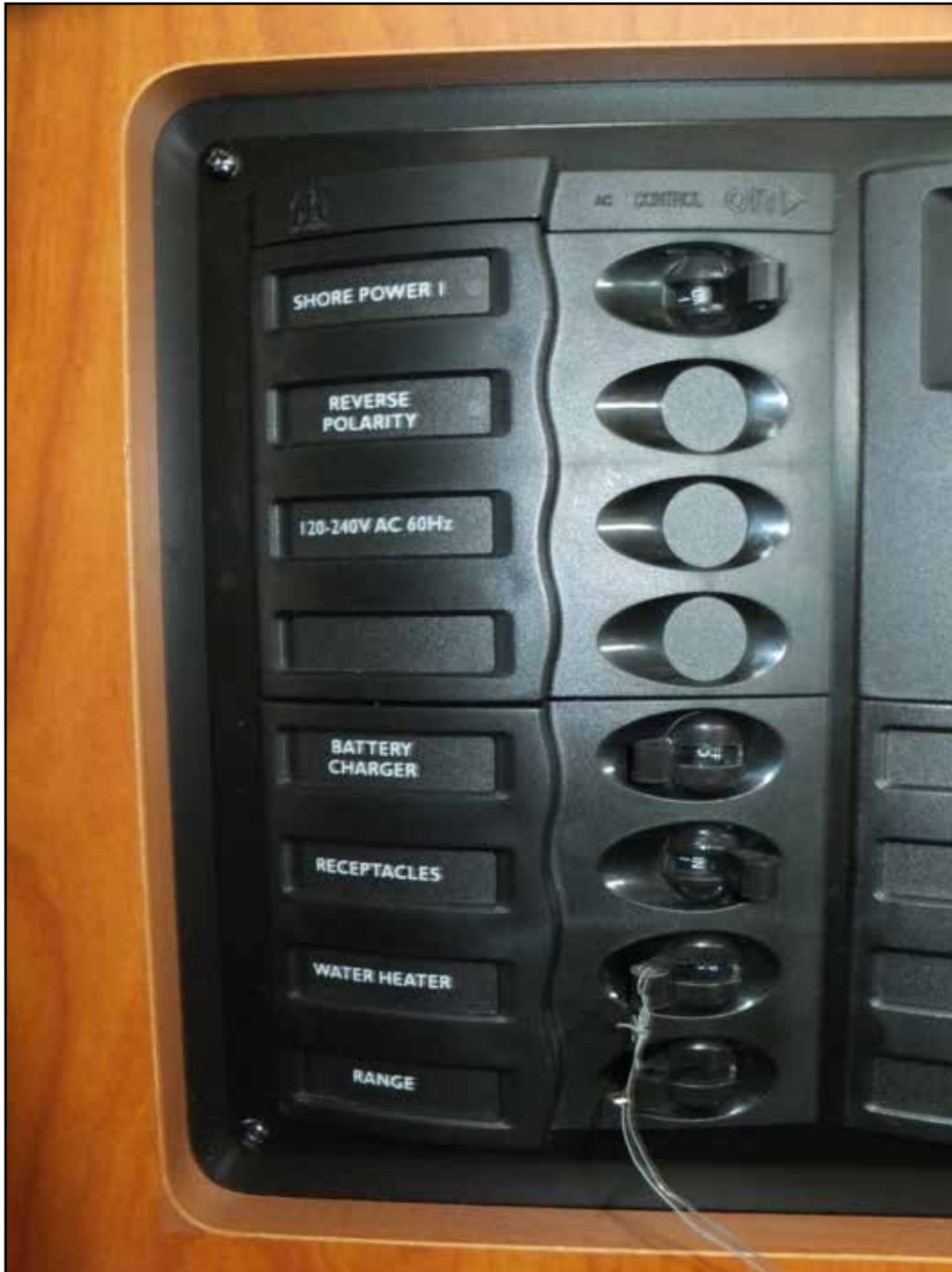
Figure 24: Battery charger/fans switch position
