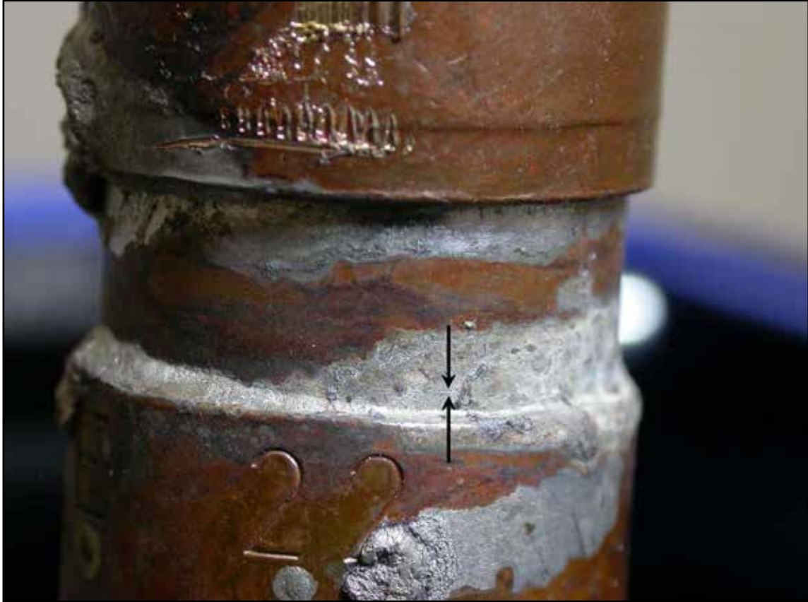
Figure 21: Previous partial failure
