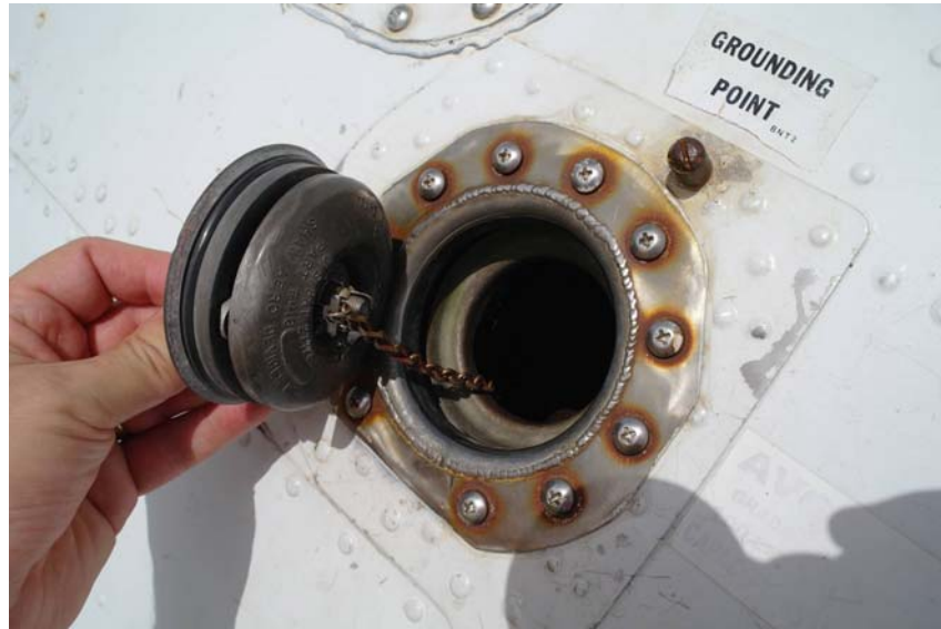
Figure 9 Left fuel tank filler neck, showing stainless steel fitting
