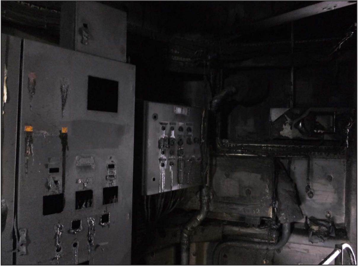
**Figure 5a:** Fire damage to thermal heater control panel
