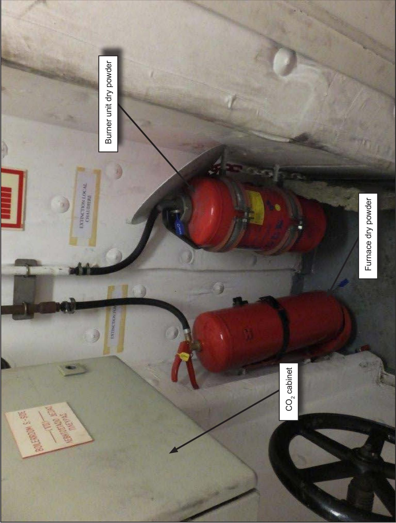
Figure 9: Photograph of fixed fire-extinguishing system control position
