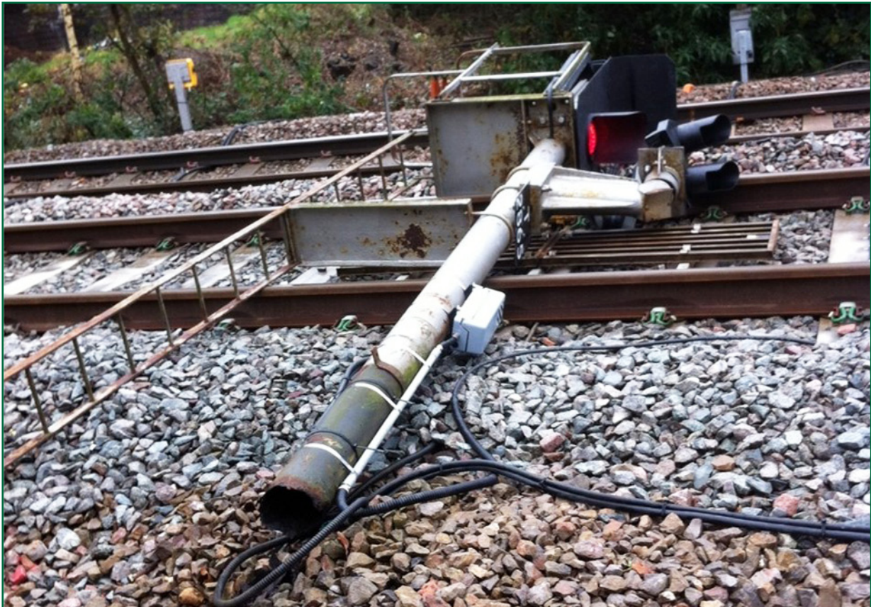
Figure 2: The fallen signal post after the accident (courtesy of Network Rail). Down Westbury line is closest to the camera, Up Westbury line is furthest away.
