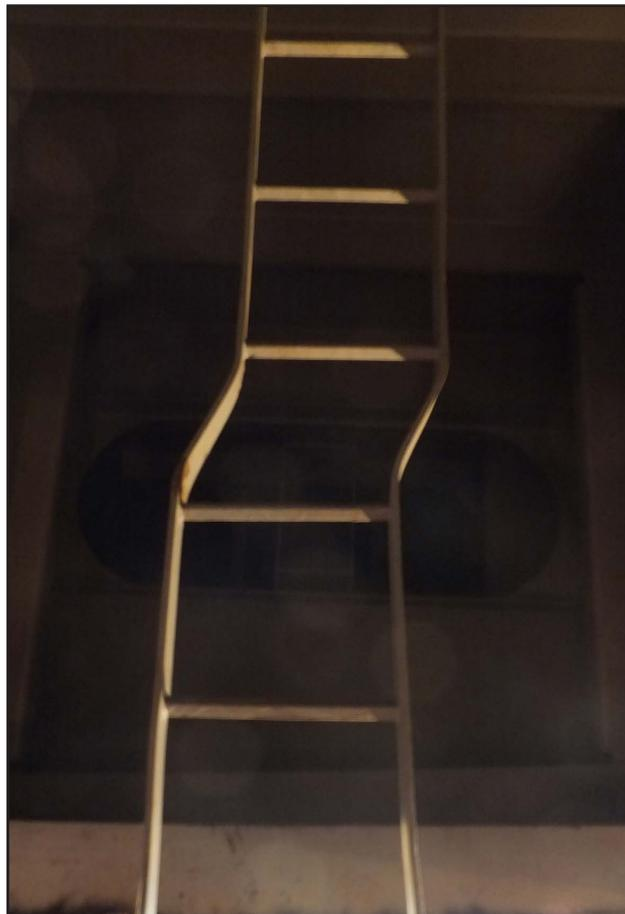
**Figure 12:** Example of internal ladder damage in a void space
