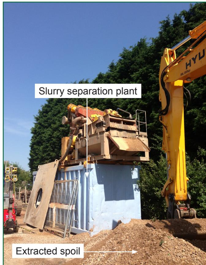
Figure D2: Slurry separation plant (image courtesy of Morgan Sindall)
