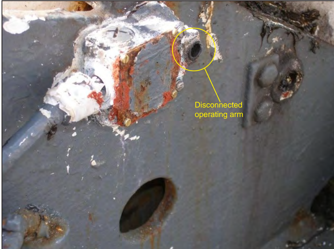
Figure 13: Broken limit switch
