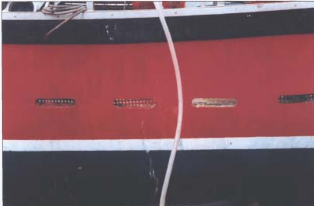
Figure 8: Plastic mesh blocking scuppers of "GORAH LASS"
