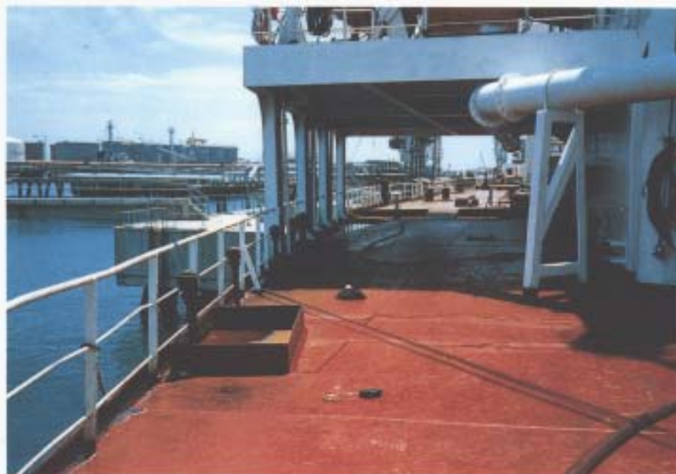
Port double bottom diesel oil tank, aft air pipe (Photographs taken on sister ships)
