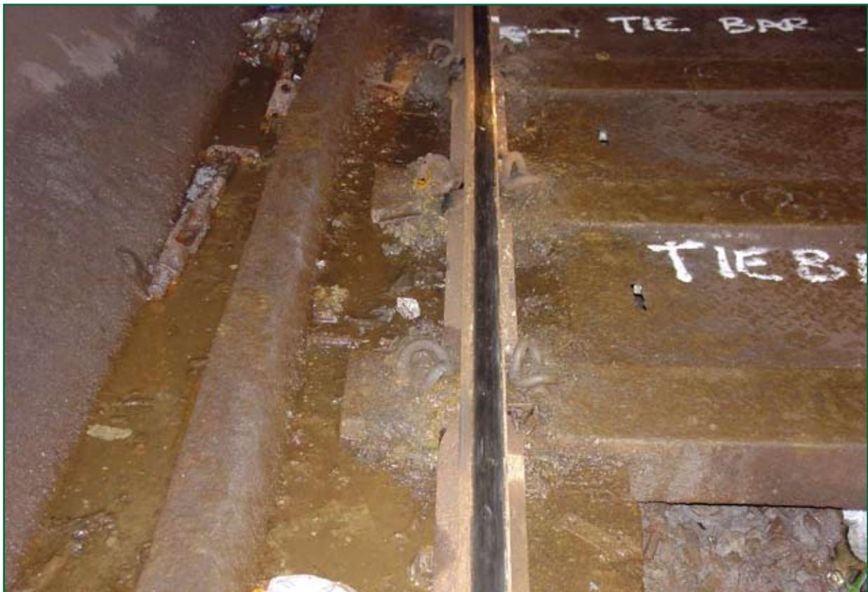
Figure 5: Showing the degree of contamination around housings and locations marked for further fitment of tie-bars
