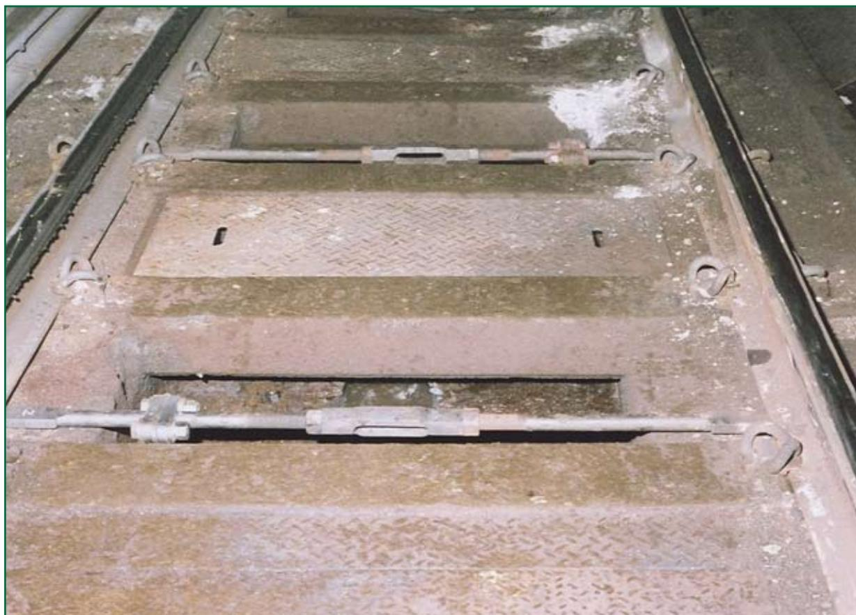
Figure 3: Tie-bars fitted to the track close to where the derailment occurred (courtesy of British Transport Police)
