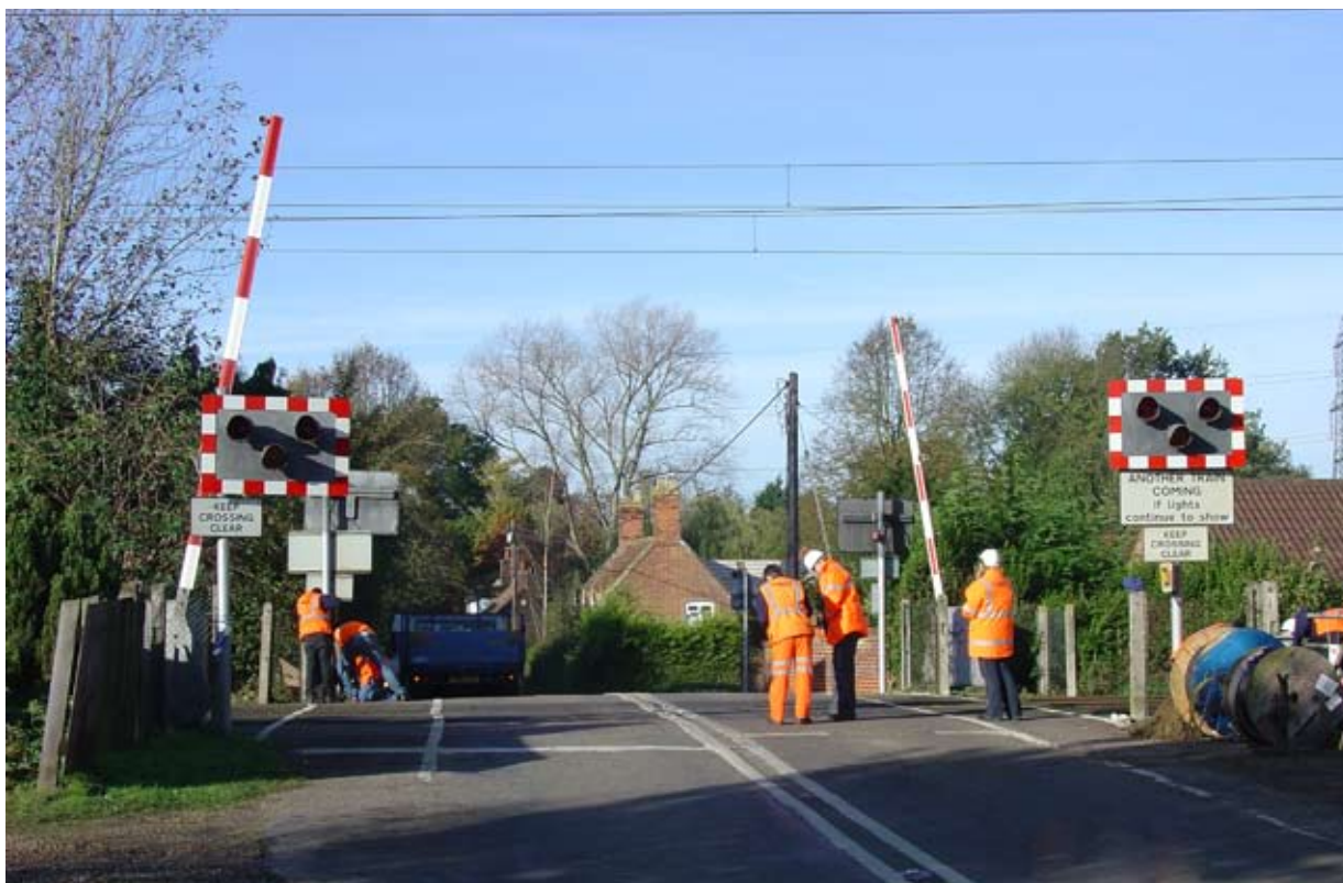
Figure 3: General view of the eastern ( Up side) approach to Swainsthorpe level crossing
