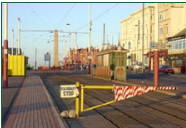
Figure 5: Temporary swinging gate at Talbot Square, looking north
