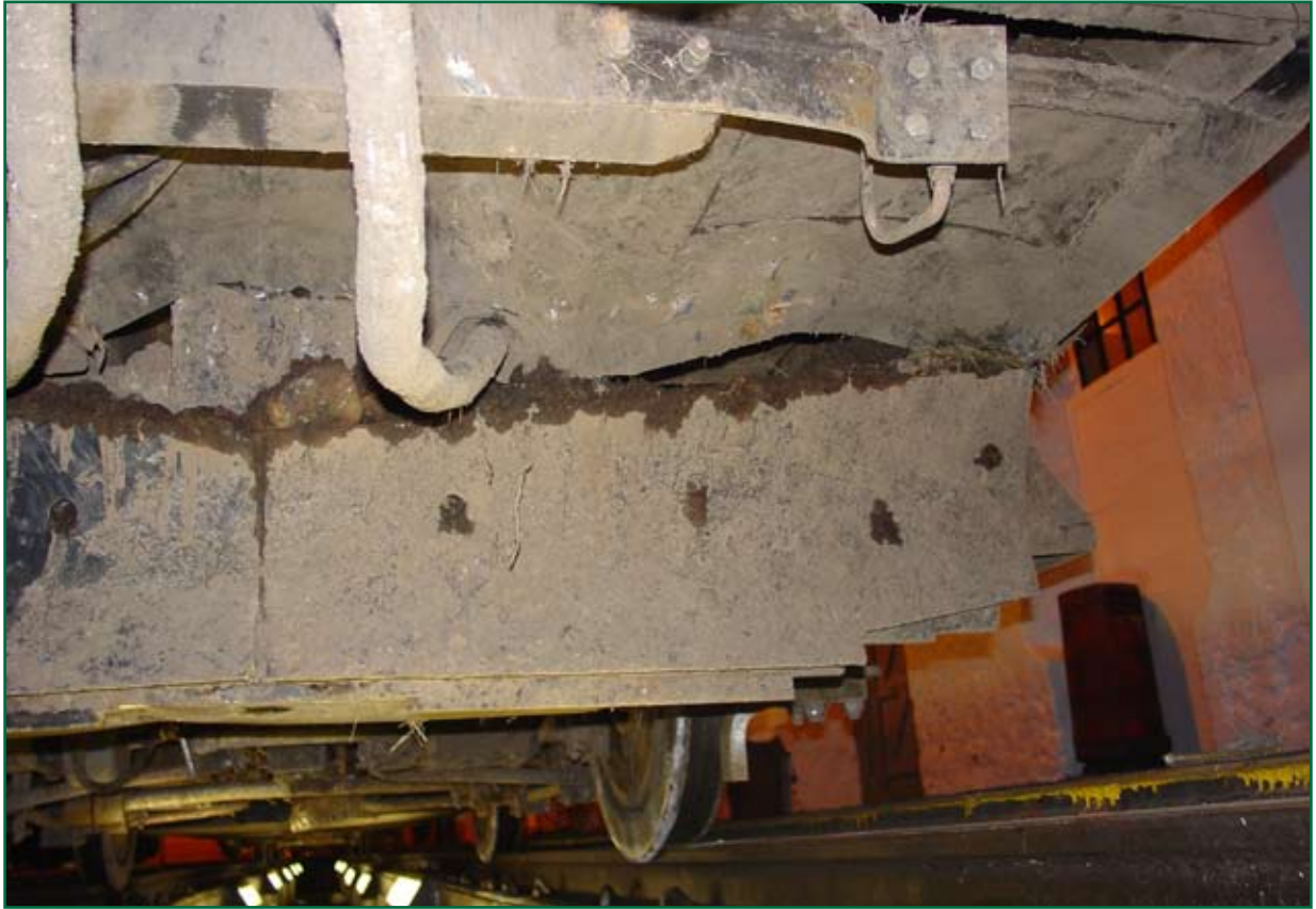
Figure 10: Underside of leading cab showing damage as a result of encountering the debris pile.
