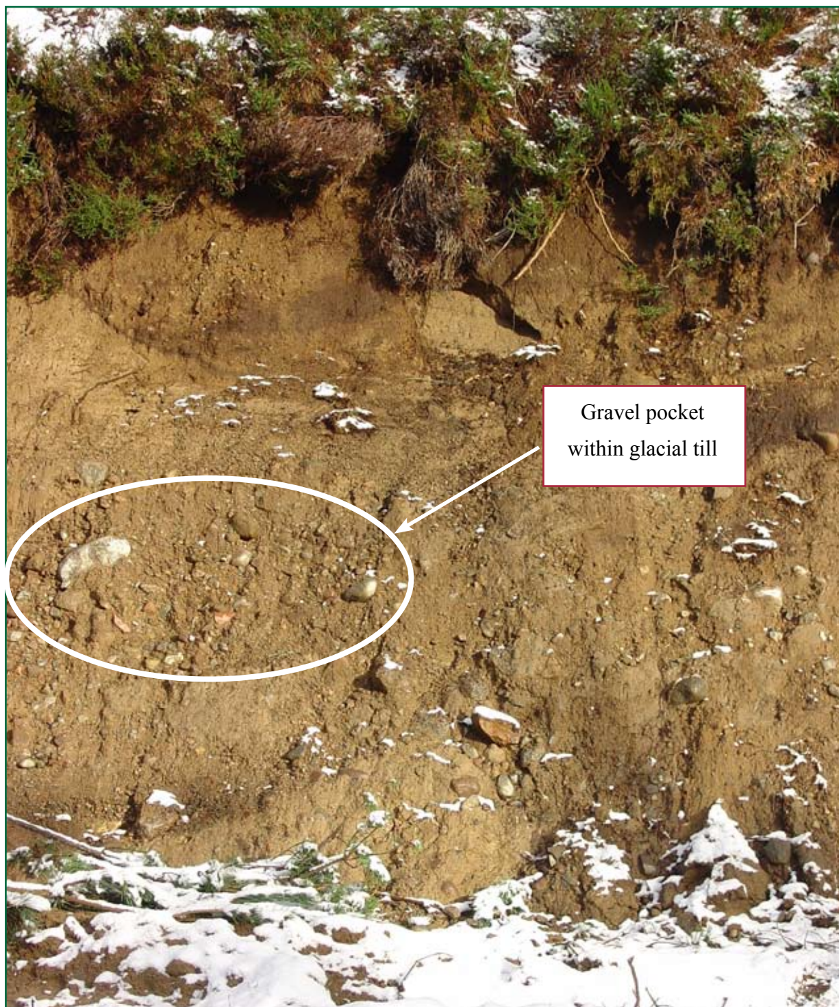
Figure 8: Backscar resulting from the landslide.
