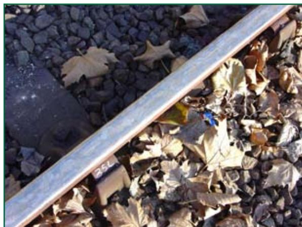
Figure 8: Track in Sudbury platform. Example of smooth rail head
