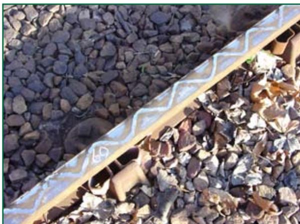
Figure 7: Track in Sudbury platform. Example of worn rumble strips and triangular rail head contact
