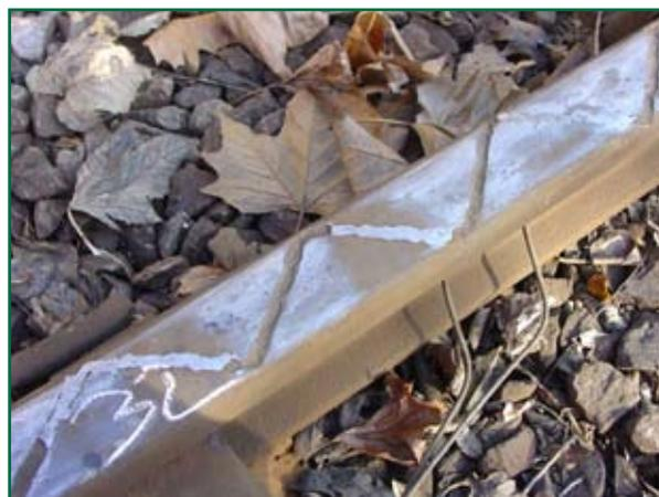
Figure 6: Track in Sudbury platform. Example of spalling of rumble strip
