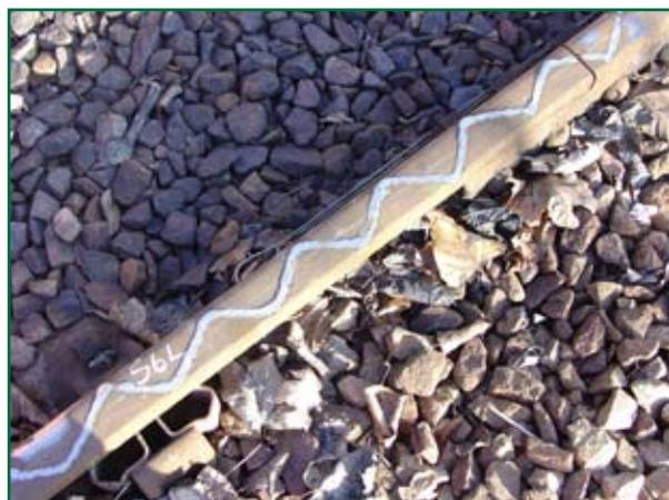
Figure 5: Track in Sudbury platform. Example of railhead with rumble strip
