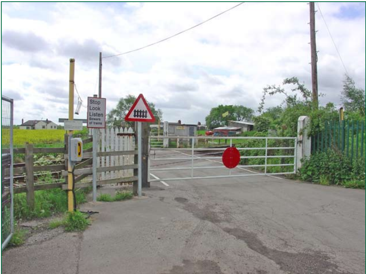
Figure 3: Crofton Old Station No.1 crossing
