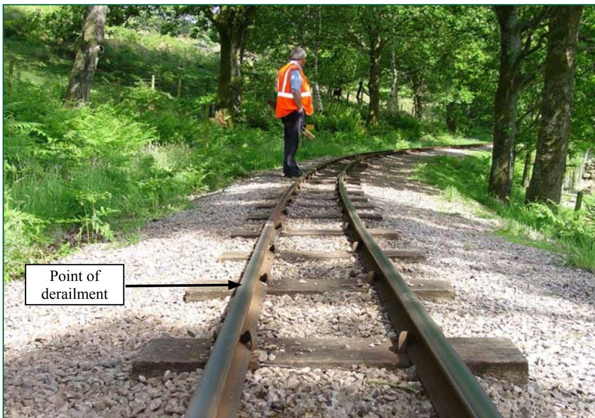
Figure 2: Site of derailment at Spout House Curve.
