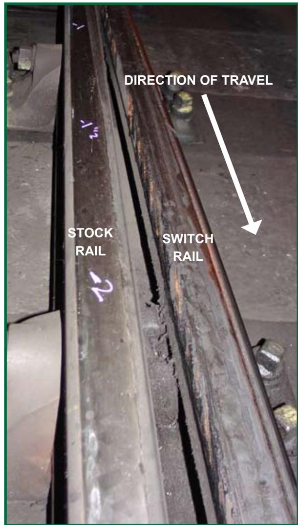
Figure 6: Right-hand switch rail showing wheel marks.
