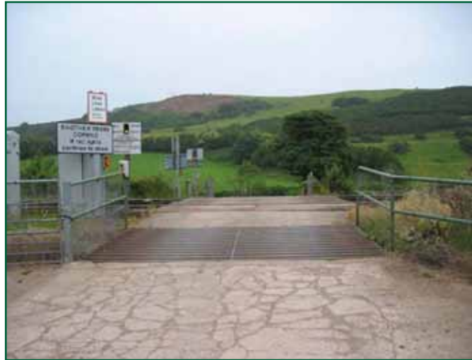
Figure 6: UWC with miniature stop lights, with gates removed (Network Rail)
