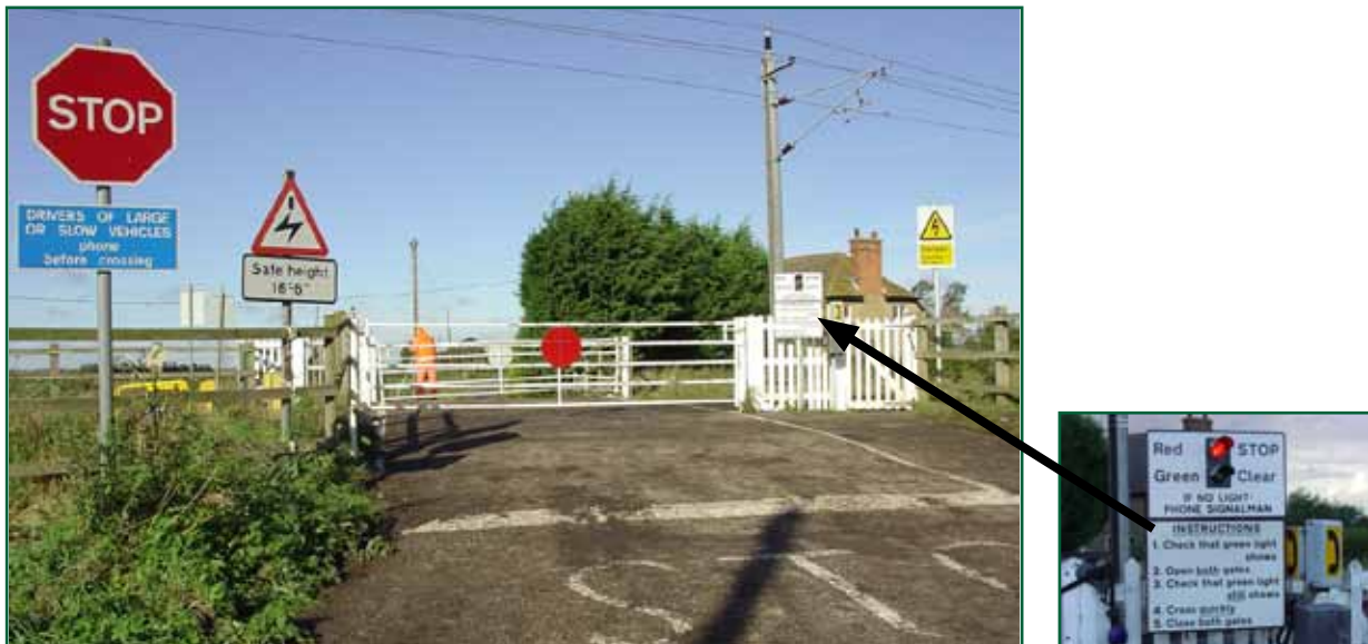
Figure 2: Example of a user worked crossing with miniature stop lights and telephones (Black Horse Drove, Cambridgeshire)
