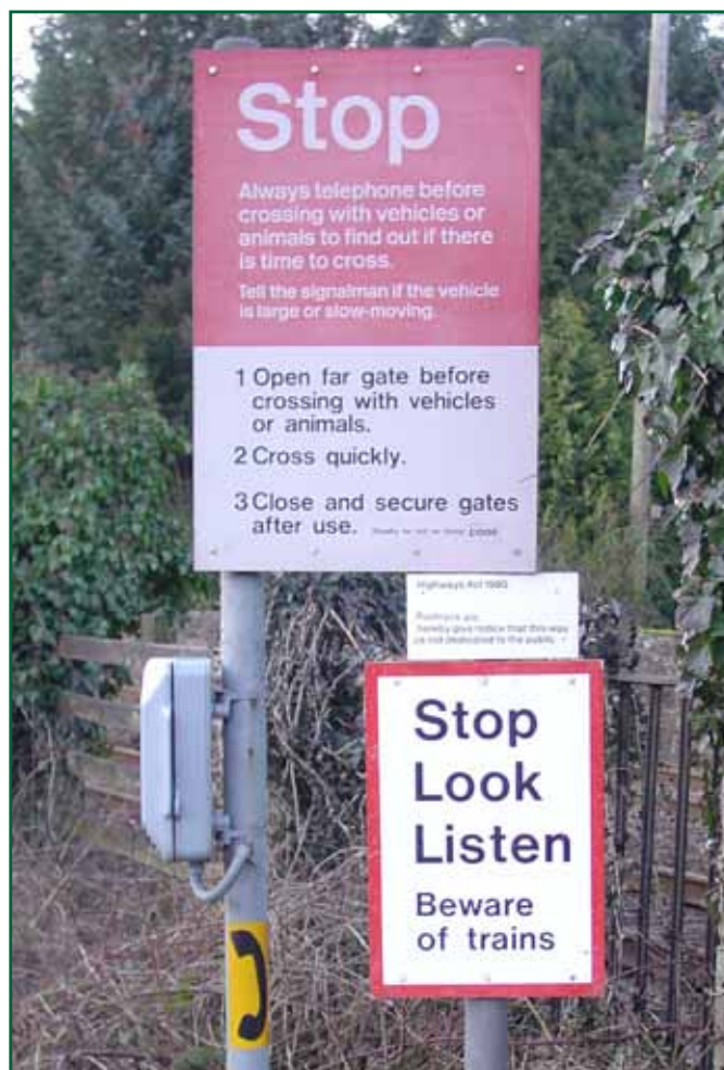
Figure 4: Signs and telephone at a UWC with a public footpath alongside it
