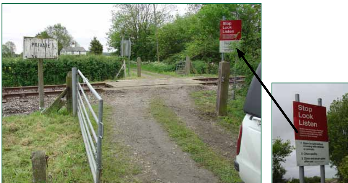
Figure 1: Example of a user worked crossing without additional protection (Bratts Blackhouse, Suffolk)
