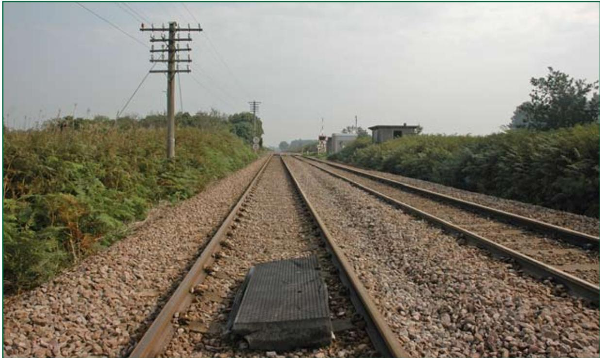
Figure 9: Dislodged HoldFast panel looking towards Croxton level crossing
