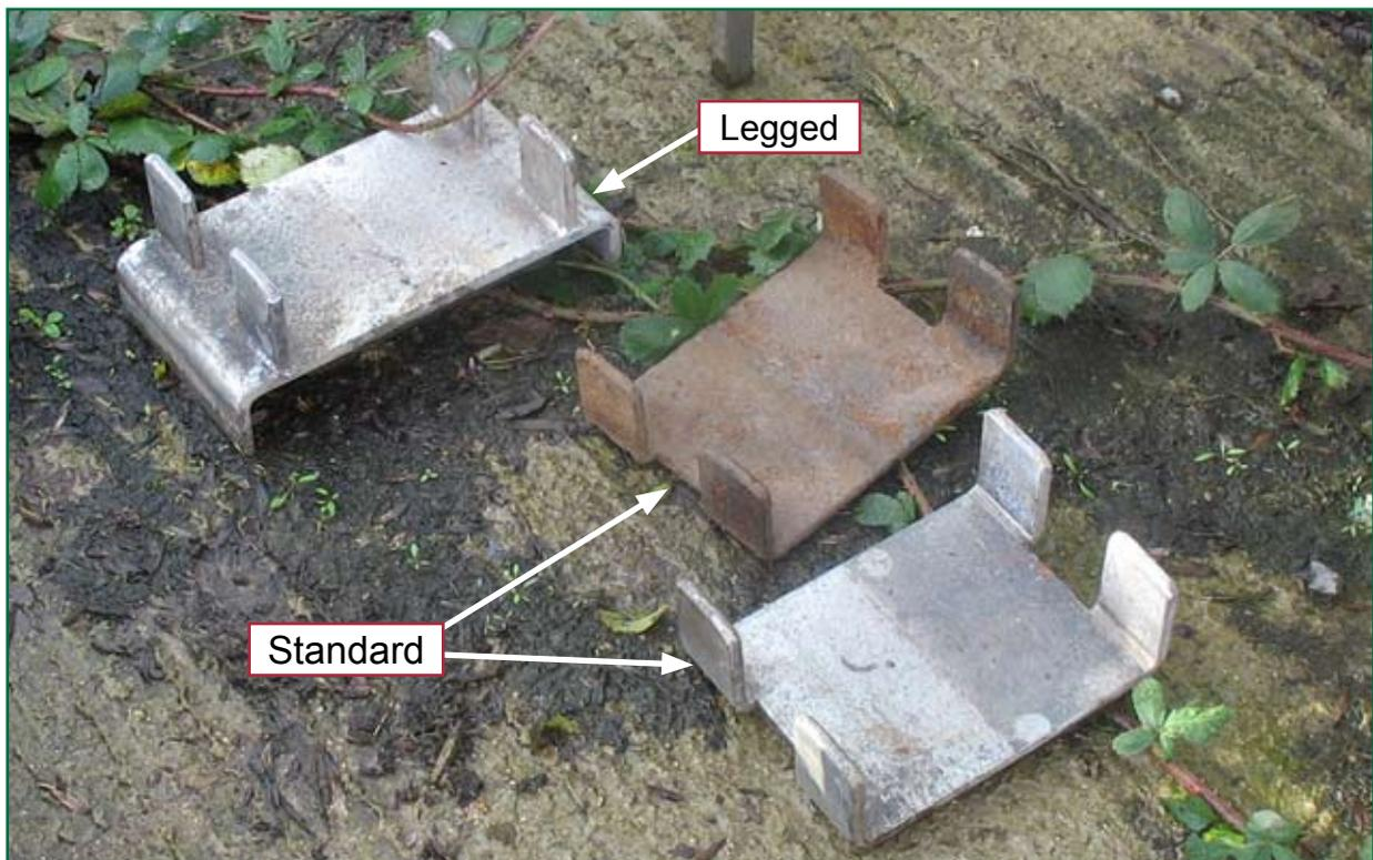
Figure 20: Legged turreted base plate (top) and two standard turreted base plates
