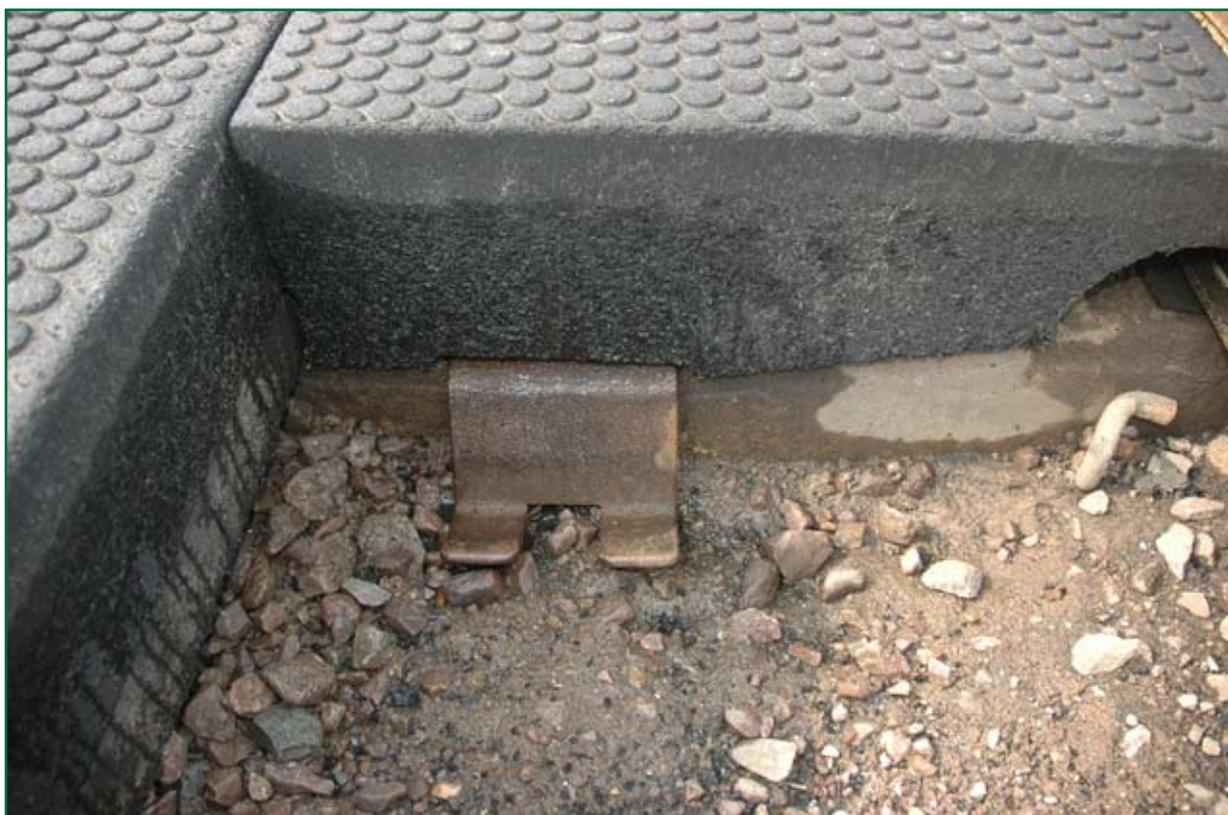
*Figure 30: Deformed base plate under Thetford end of dislodged panel B4*
