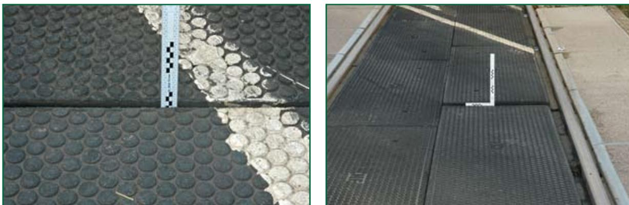
Figure 24: Vertical differences between upper surfaces of adjacent panels at Croxton
