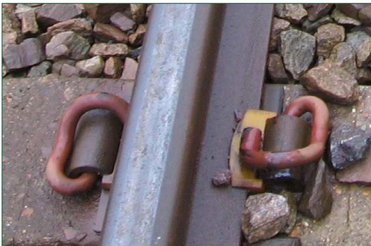
Figure 22: Pandrol rail clip and insulators
