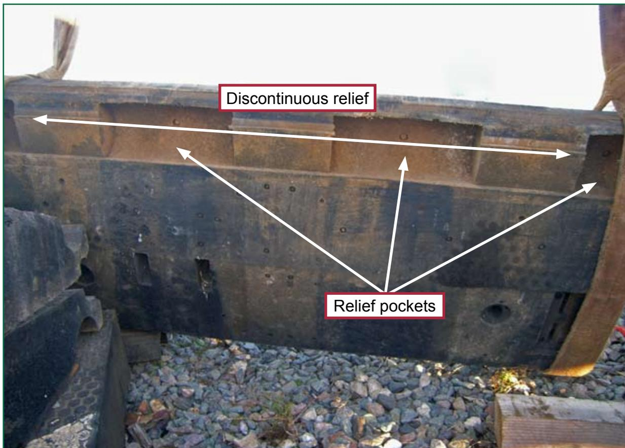
Figure 14: Discontinuous relief area on HoldFast panel underside
