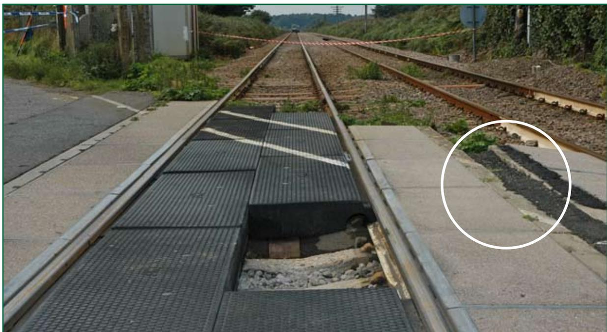
Figure 4: Raised six foot Bowmac edge beams (circled)
