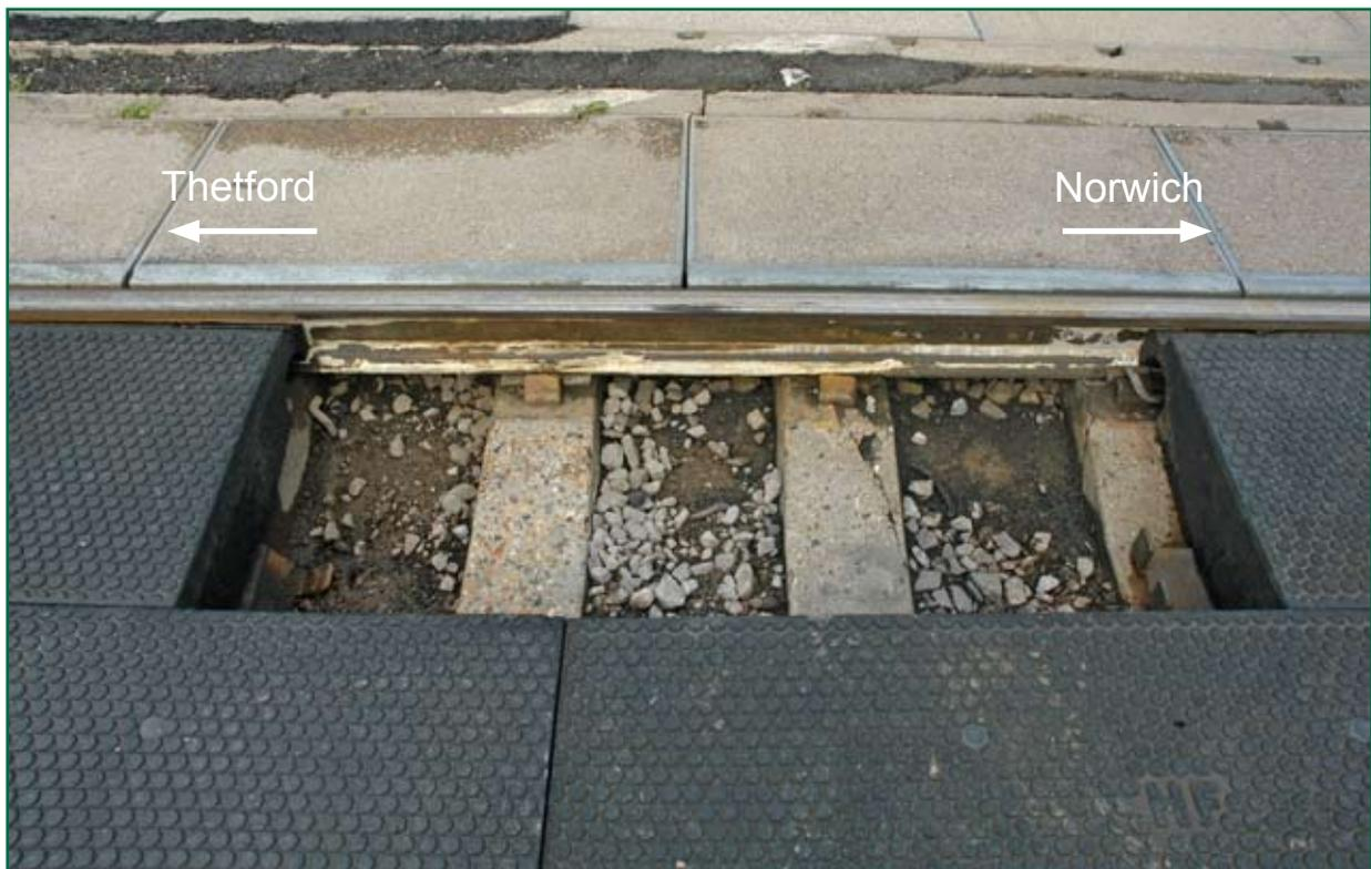
Figure 23: Six foot rail and sleepers under dislodged panel B4
