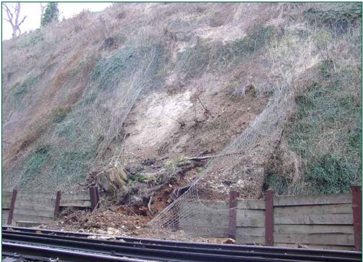
*Figure 9: Hooley cutting showing the landslide*
