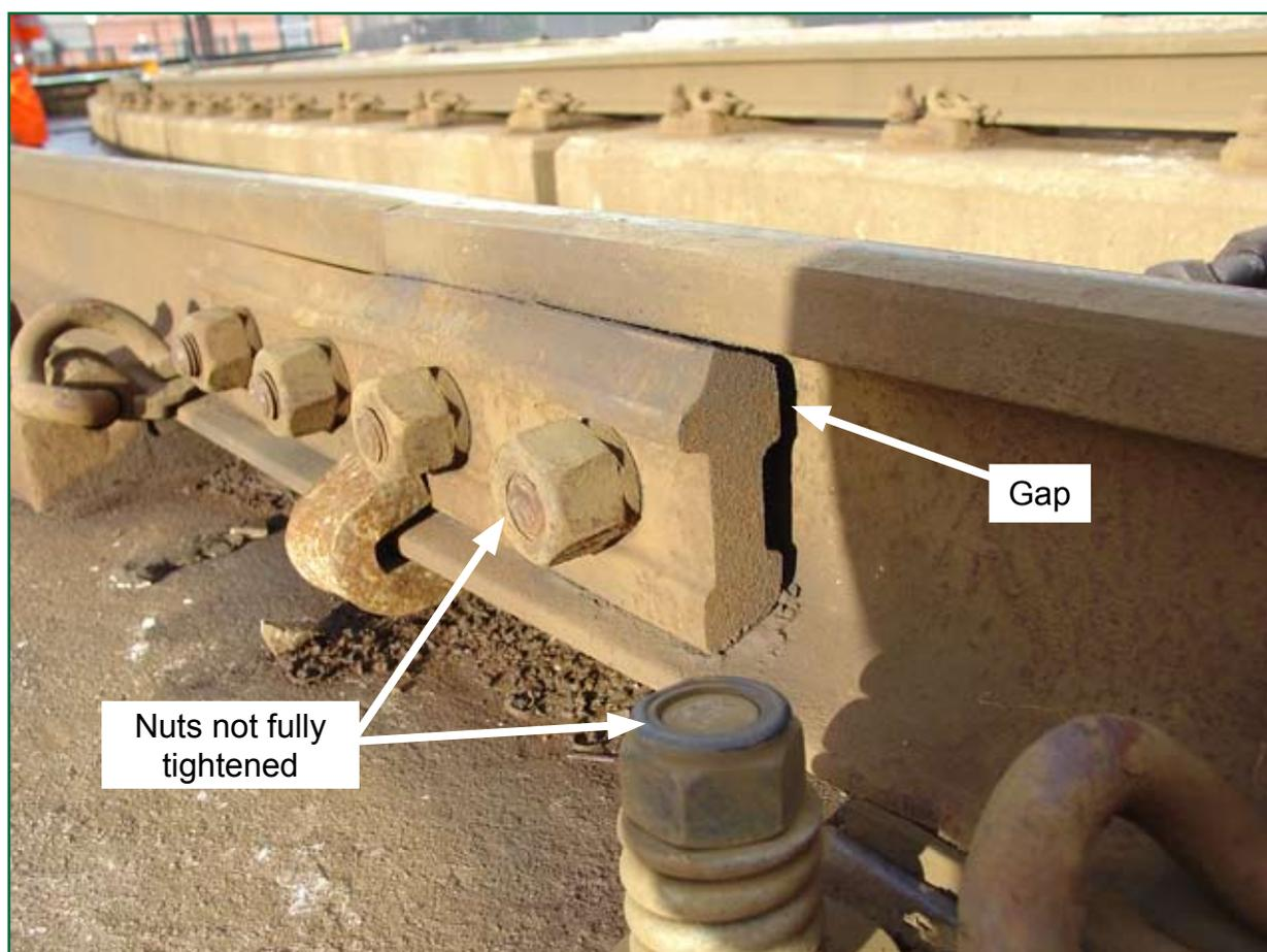
Figure 6: Rail joint in six-foot rail at point of derailment
