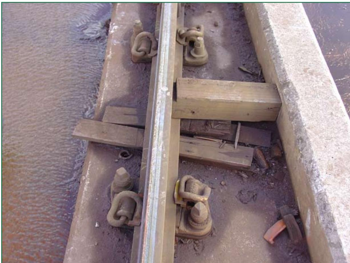
Figure 7: Timber propping six-foot rail against concrete upstand
