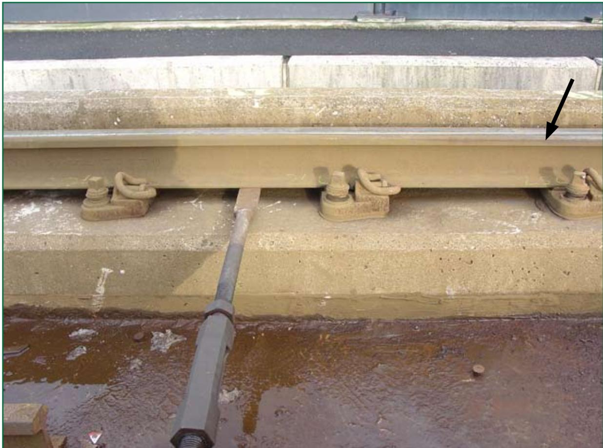
Figure 4: (left) side rail, showing wheel drop-in mark (arrowed)
