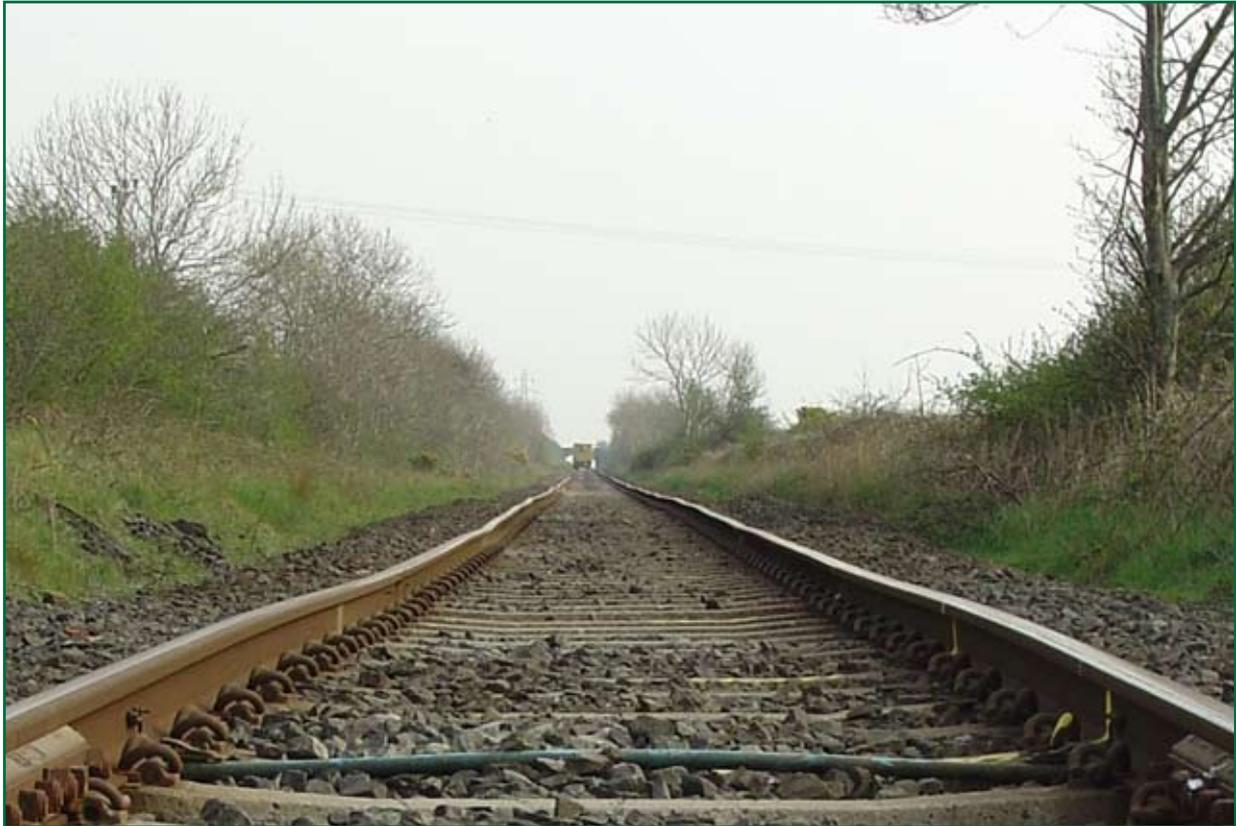
*Figure 5: Track near point of derailment, showing cyclic top*
