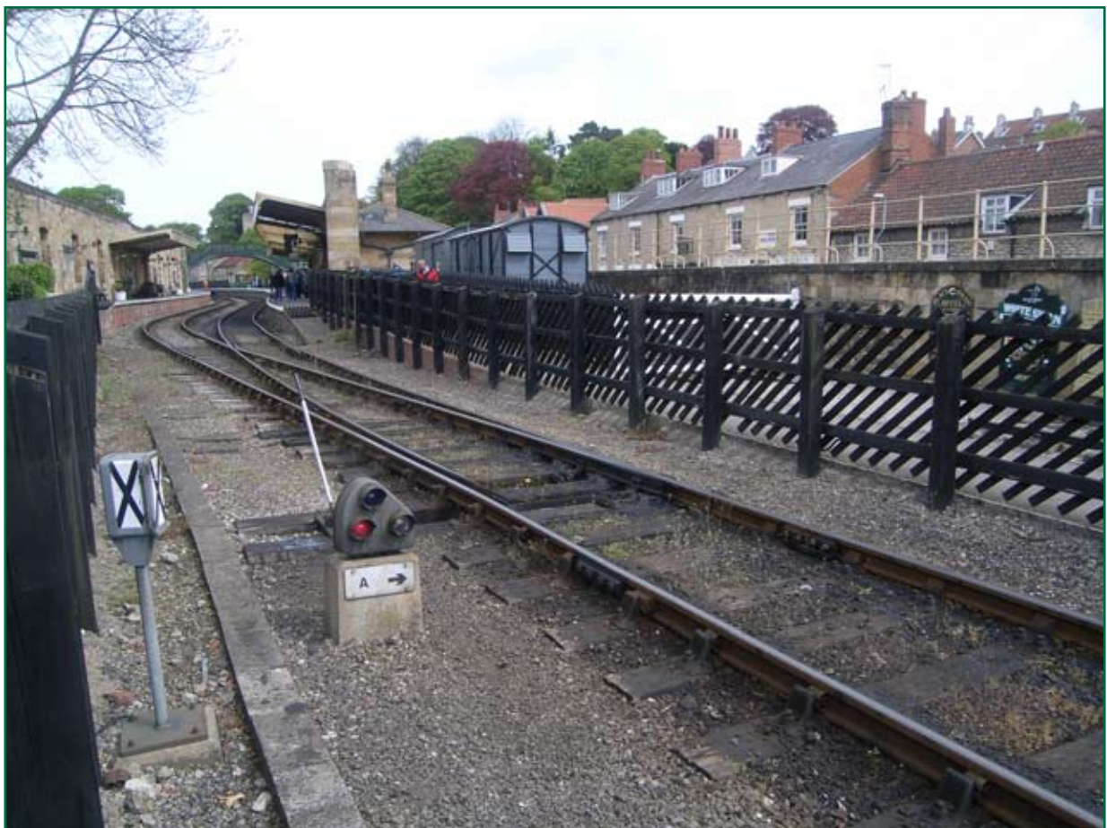
Figure 4: Points lever and ground signal at Pickering south
