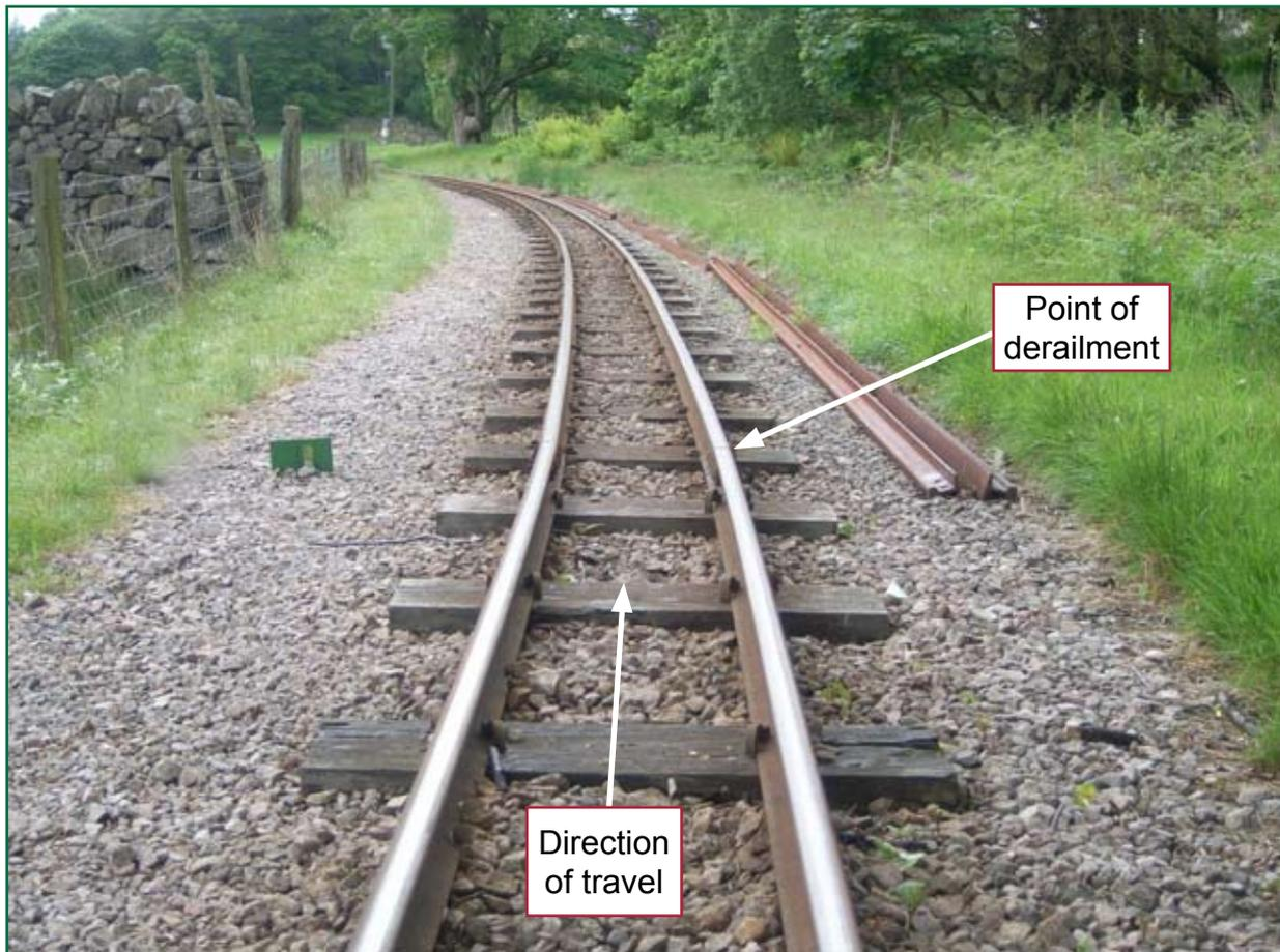
Figure 2: Site of derailment at Hollin How
