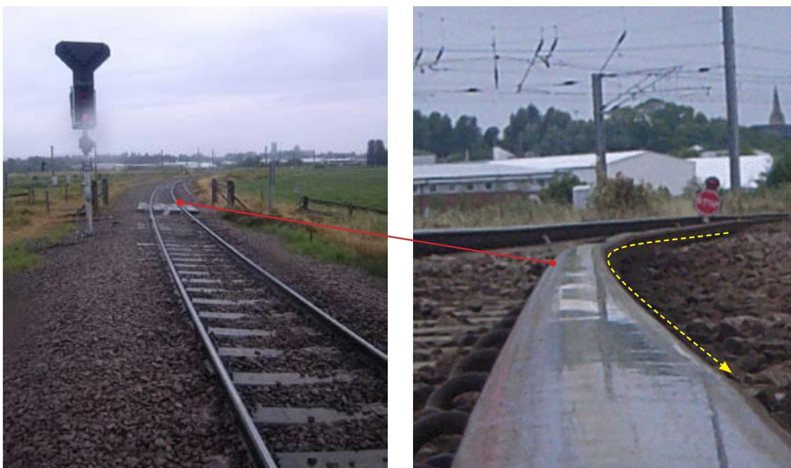
Figures 8 (left) showing view of track towards Ely with right high rail on left and low left rail on right. Figure 9 (right) view of track towards Ely showing low left rail (foreground) and high right rail (background) at the point of derailment
