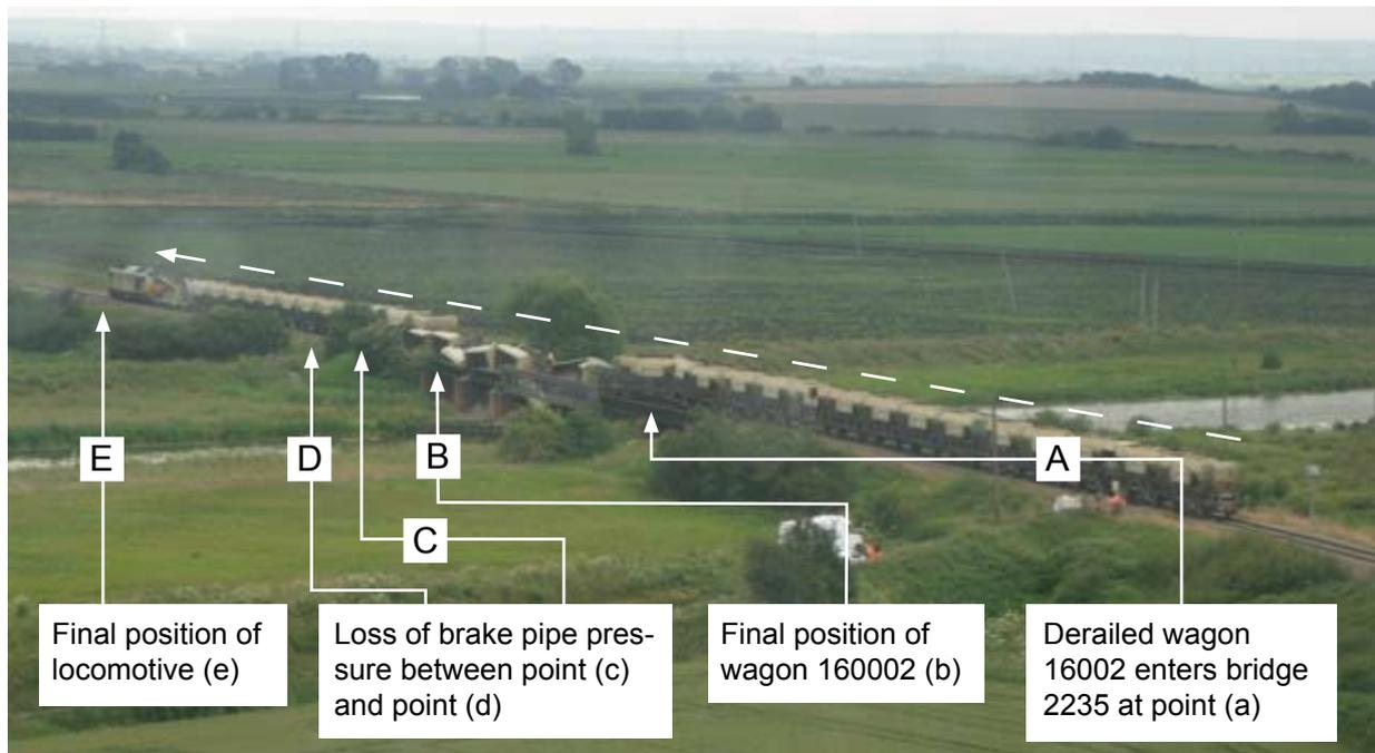
Figure 10: Image showing final position of train 6L58 on bridge 2235 (aerial images are shown at appendix E)
