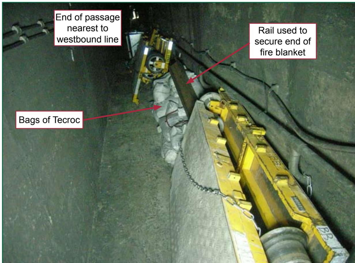
Figure 8: Equipment stored in the cross passage as found immediately following the derailment and viewed from end closest to the eastbound track
