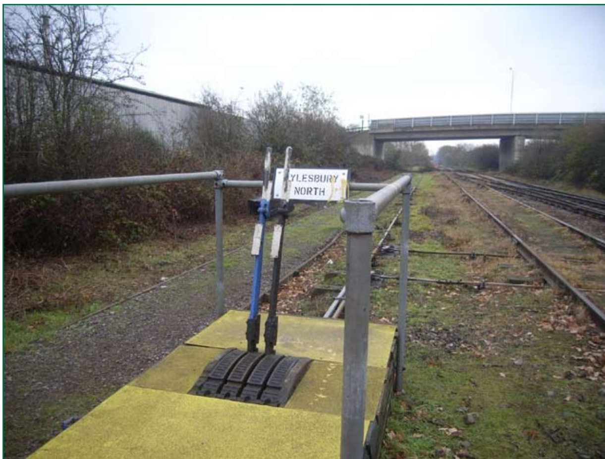
Figure 3: Aylesbury north ground frame
