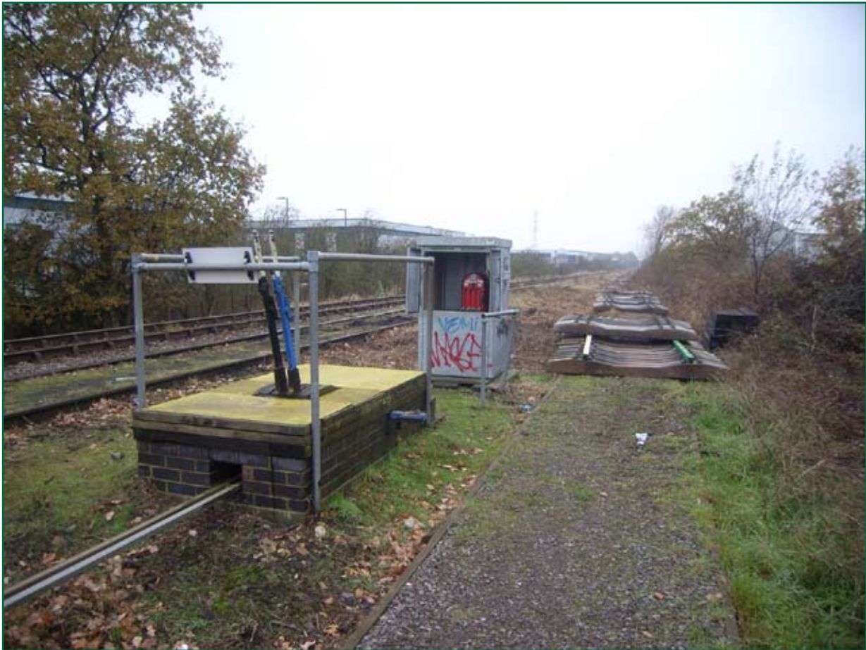
Figure 7: Ground frame and token instrument at Aylesbury north
