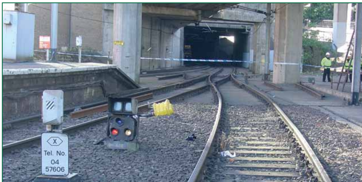
Figure 4: Photograph of the start of the slab track section at Exhibition Centre station, looking towards Anderston and the western portal of Stobcross Tunnel. This is shown as location 4 on Figure 3
