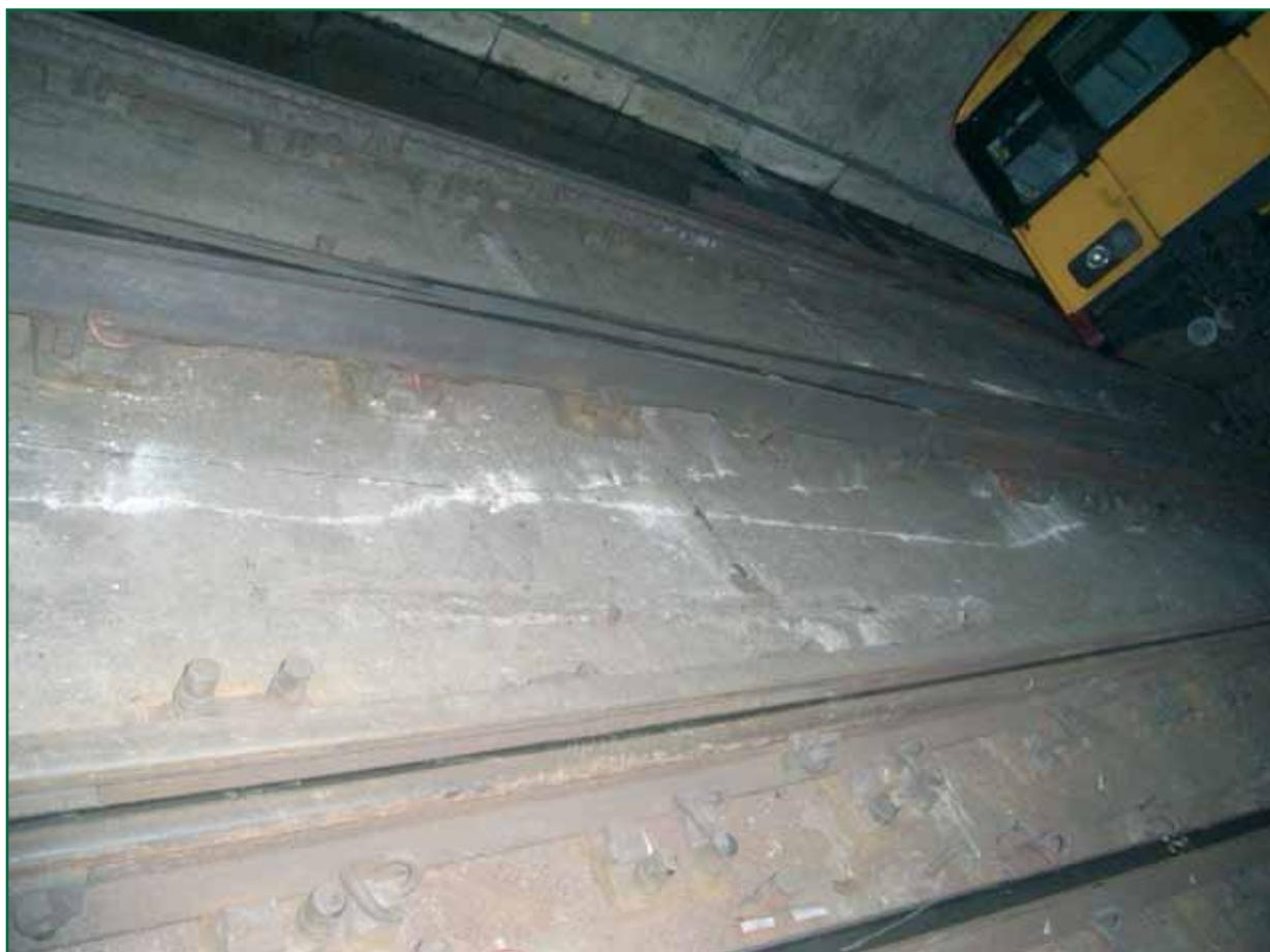
*Figure 18: Slab track with fixtures connected directly to the base concrete. Also scores made by the flanges of the derailed wheels.*
