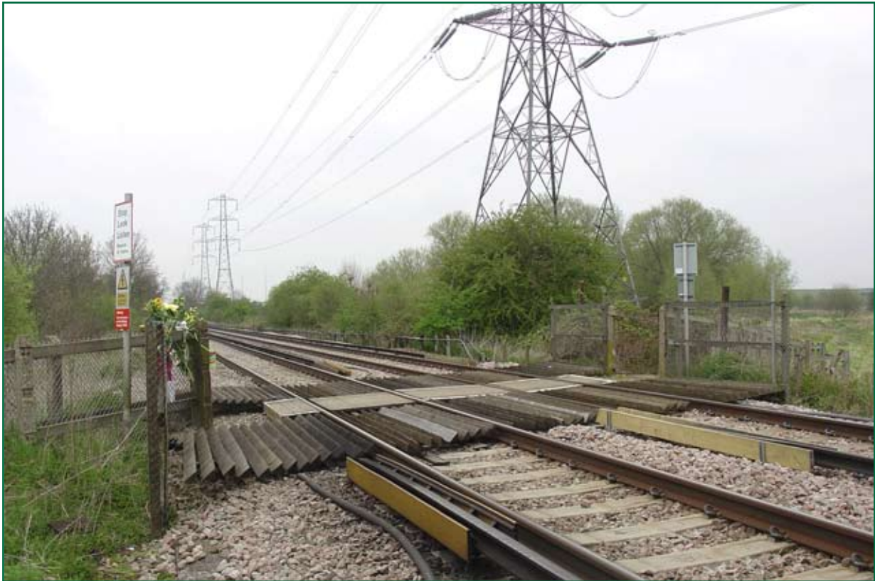
Figure 2: Moor Lane crossing from the south-east
