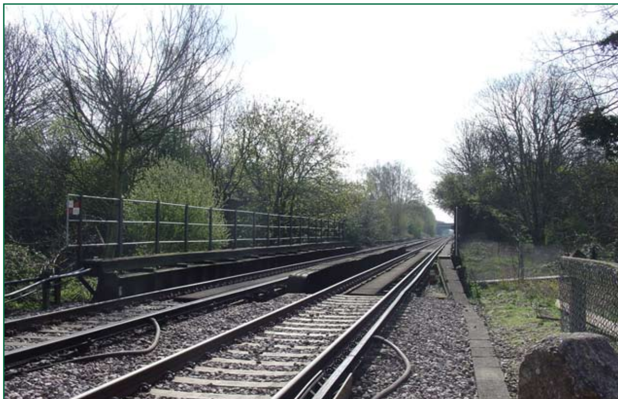
Figure 6: View south-east from end of approach path
