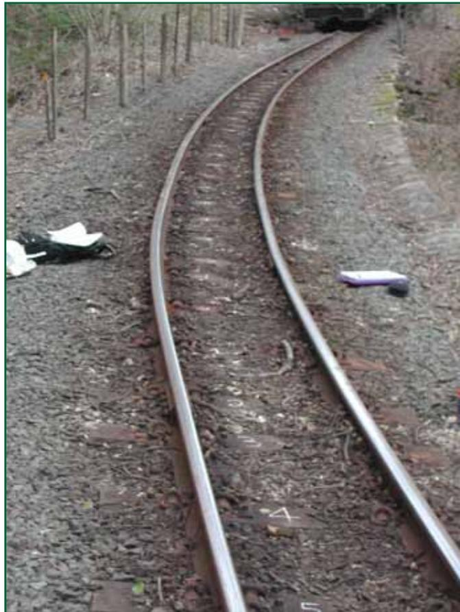
*Figure 2: Gysgfa curve following the derailment*
