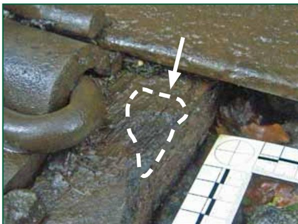
Figure 7: Timber surface adjacent to baseplate - damaged surface shown arrowed
