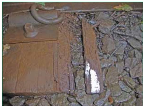
Figure 8: Timber sleeper affected by decay
