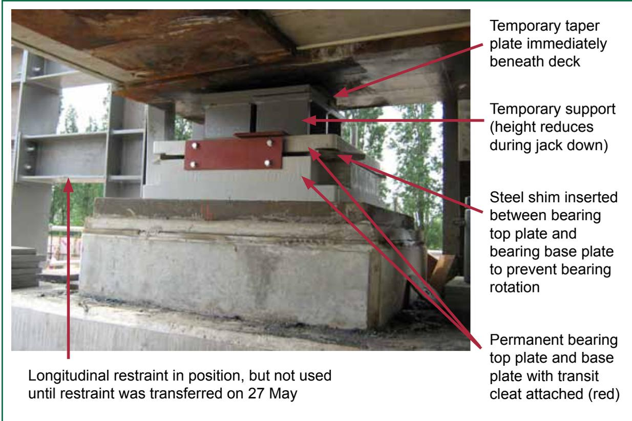
Figure 20: Photograph of south-east bearing during jack down (photo TfL).
