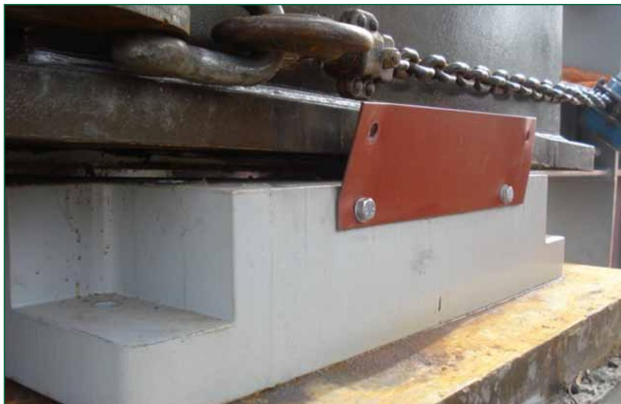
*Figure 23: Failed transit cleat on south-east bearing (photograph BB-CJV)*
