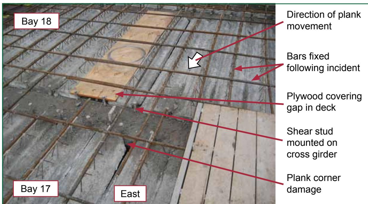
Figure 10: Photograph showing damage to deck (photograph TfL)
