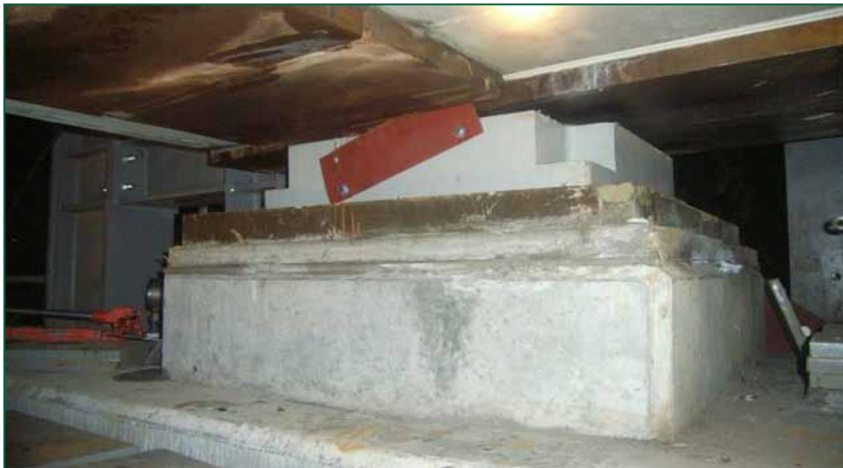
*Figure 22: South-east bearing following collapse showing a failed transit cleat.*
