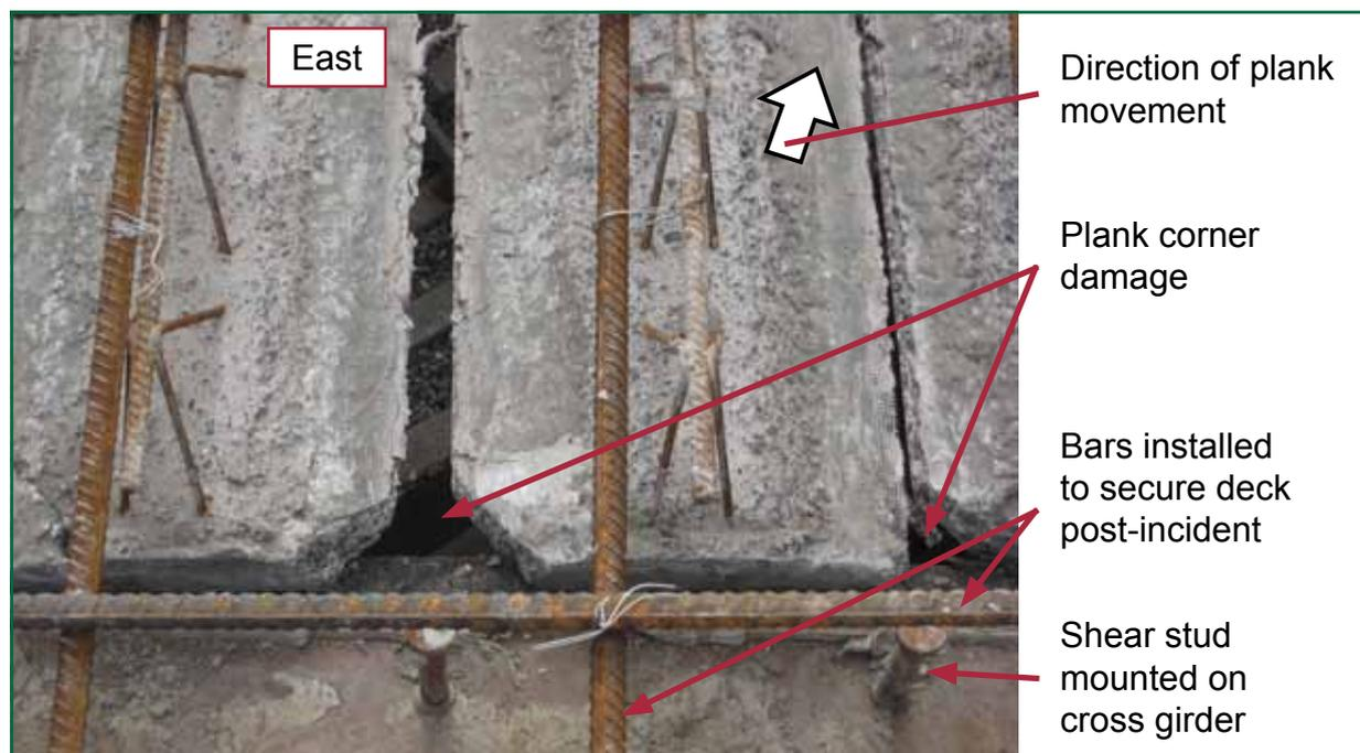
Figure 11: Photograph of damage to permanent formwork planks. The track is visible through the gap (Photograph TfL)
