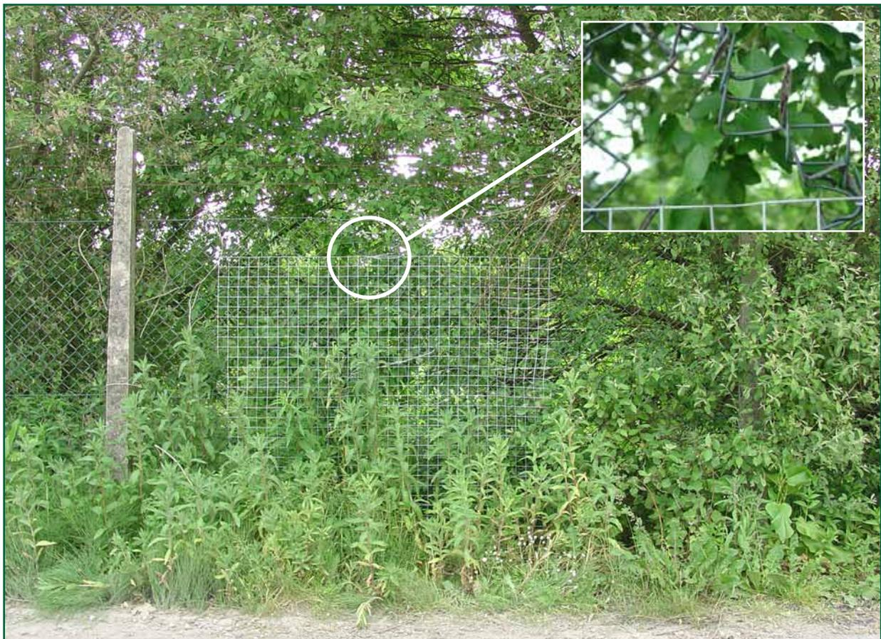
Figure 19: The repair to the hole in the fence
