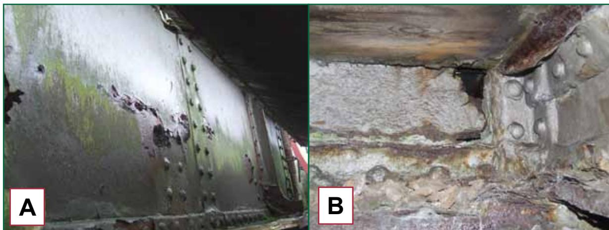
Figure 23: Photographs of web corrosion from the Inspection for Assessment undertaken 27 November 2007 (photographs courtesy of Network Rail)
