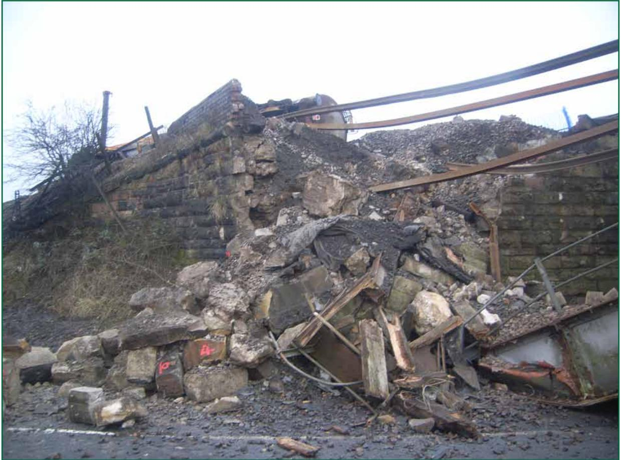
*Figure F4: Photograph of debris from failed south abutment*
