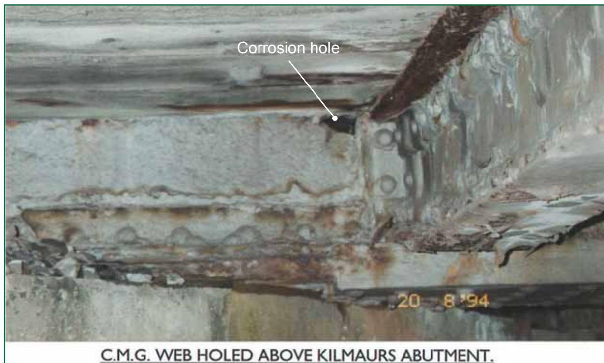
Figure 21: The web plate corrosion hole at the south end of the centre main girder that was illustrated in the 1994 Assessment report (photograph courtesy of Network Rail)
