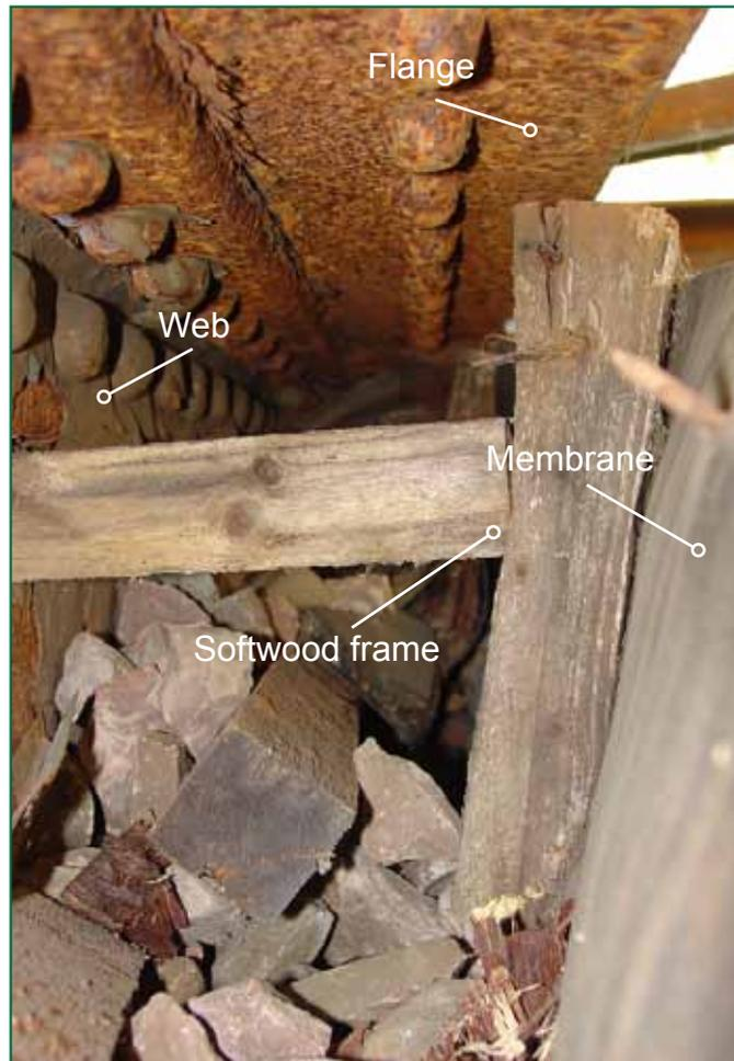
Figure 18: Accumulated ballast and debris found behind the waterproof membrane of the centre main girder
