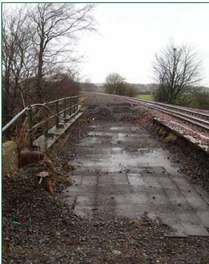
*Figure F3: Site photograph of the west deck after the ballast was removed on 16-17 January 2009 (photograph courtesy of Network Rail)*
