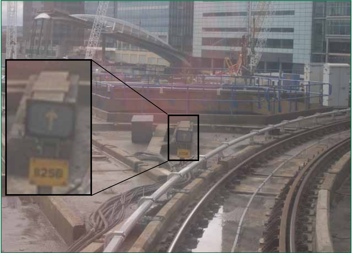
Figure 10: 1125B point position indicator displaying a white arrow and viewed from a stationary train in approximately the same position as train LEW109 was after emergency braking
