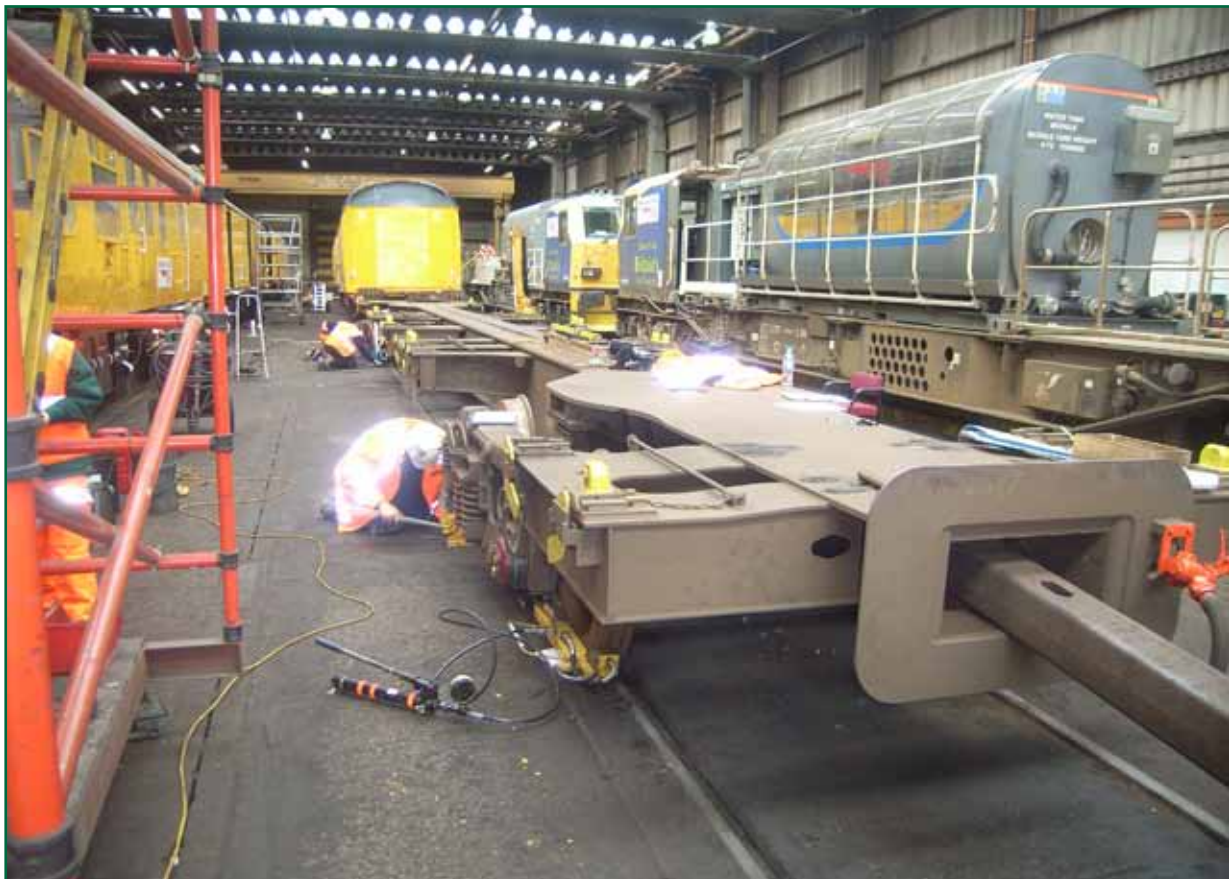
Figure 2: Wagon which derailed showing bar coupling to adjacent wagon
