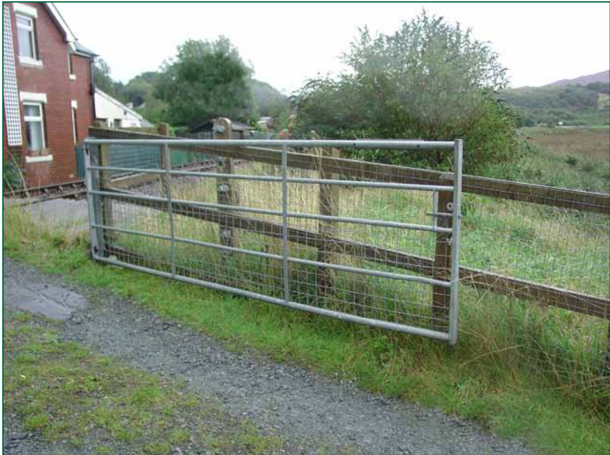
Figure 4: Restricted view from road on the south side of crossing in the direction of Penrhyndeudraeth station
