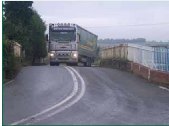
Figure 7: Southbound vehicle straddling centre white lines due to sharply curved road alignment
