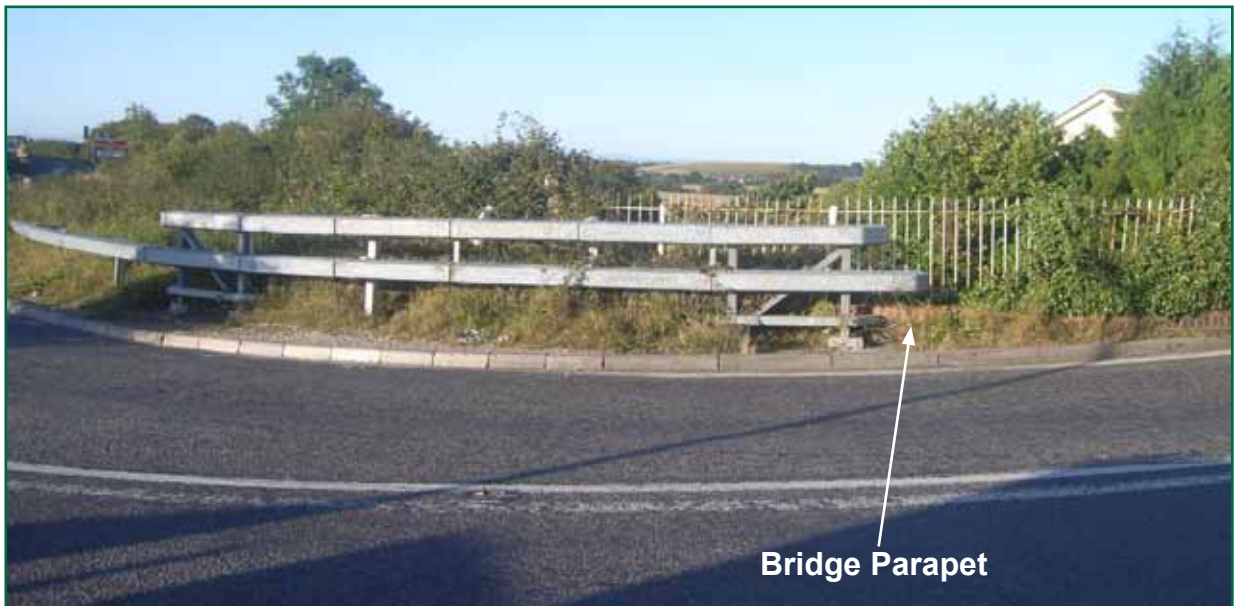
Figure 5: Steel crash barrier installed at the south-east corner of the bridge
