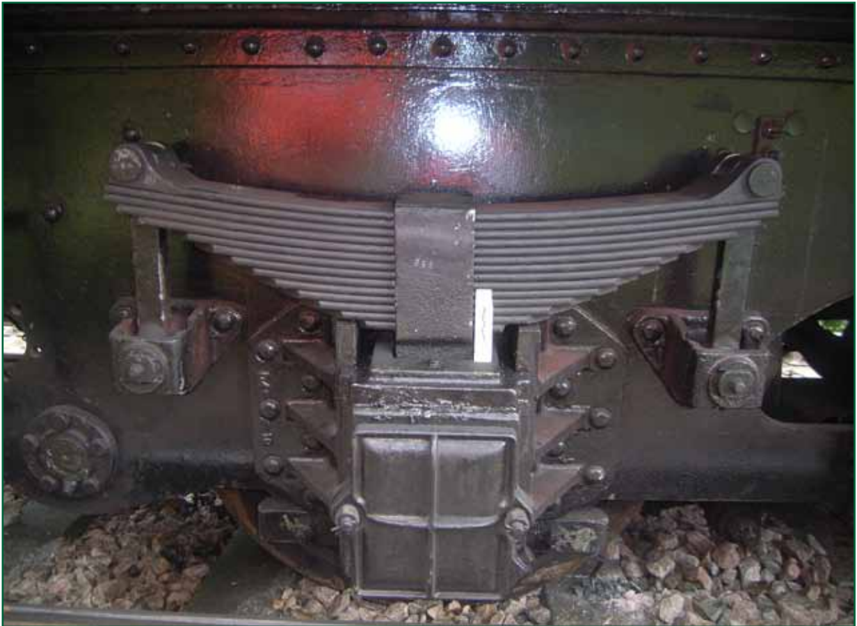
Figure 4: New spring fitted to leading left side of tender
