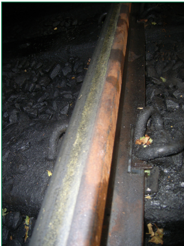
Figure 2: Contamination on the rail-head at the south end of the station
