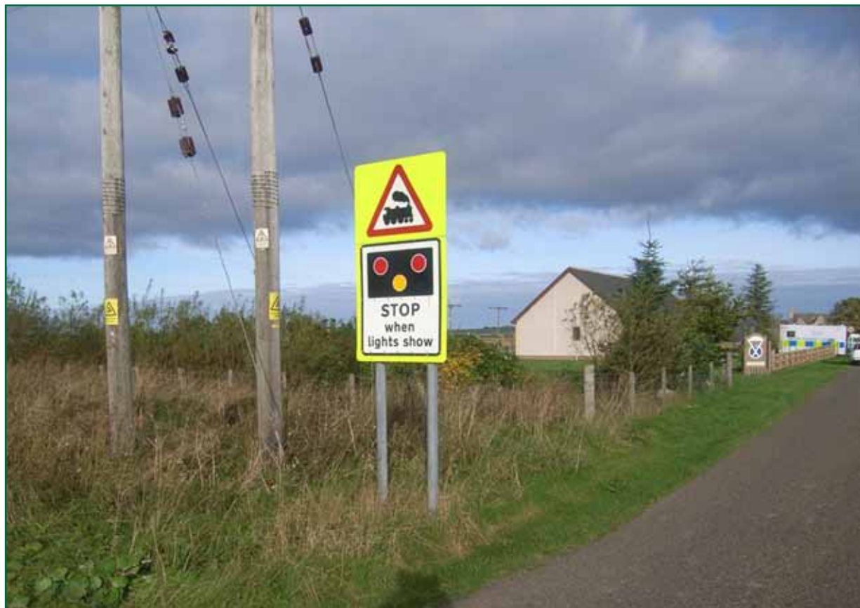
Figure 4: Signage on the approach to Halkirk level crossing
