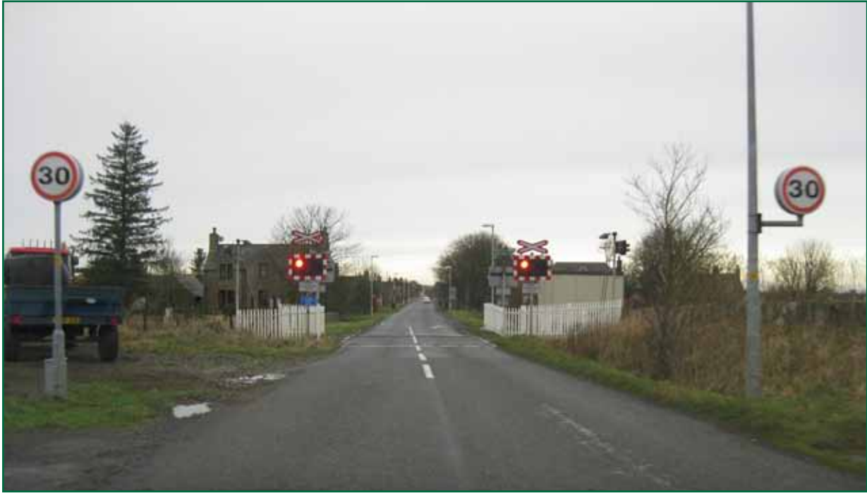
Figure 9: the 30 mph signs at Halkirk crossing (taken after the accident and the renewal of the road lights to the LED type)
