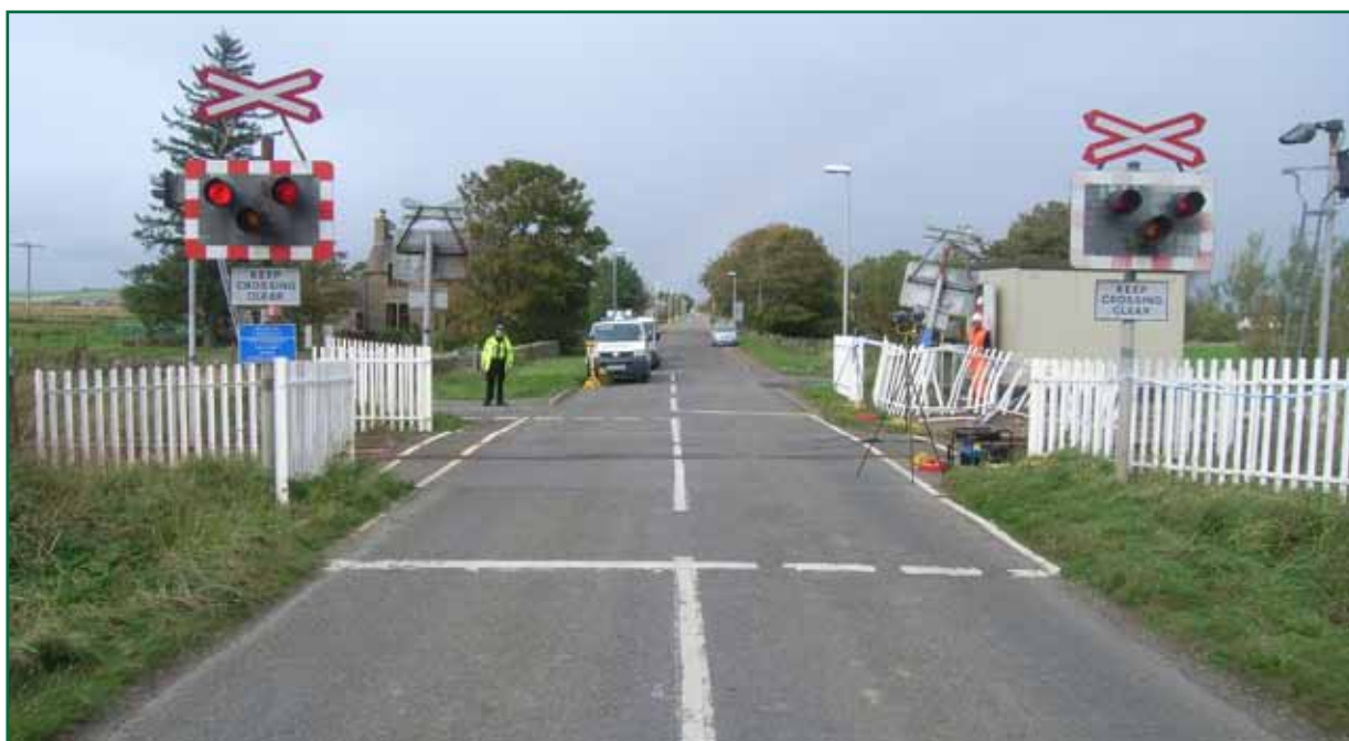
Figure 3: Halkirk level crossing from the south
