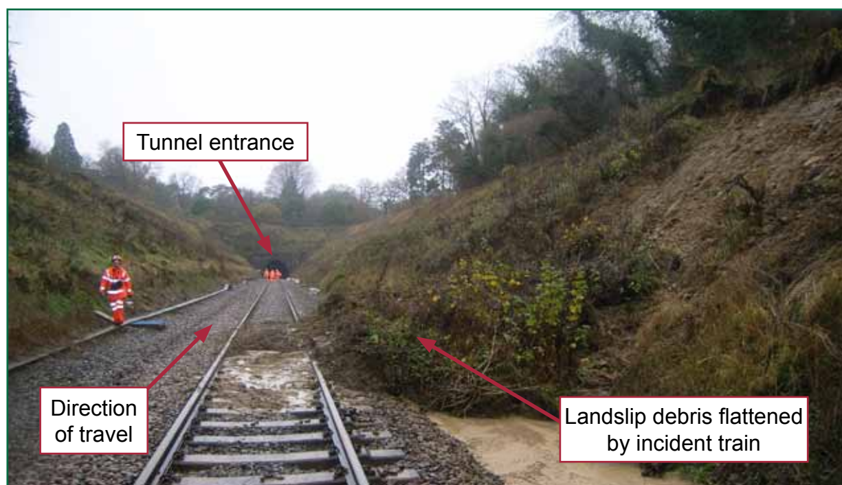
Figure 3: Track level view of accident site
