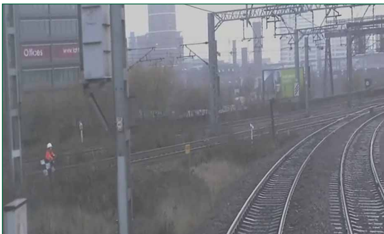
Figure 4: The west-facing lookout viewed from the Leeds-bound train
