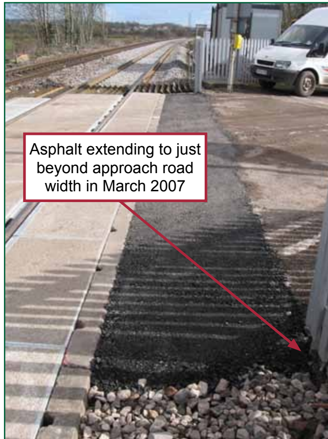
Figure 10: The asphalt section following the work in March 2007 (photograph courtesy of Network Rail)
