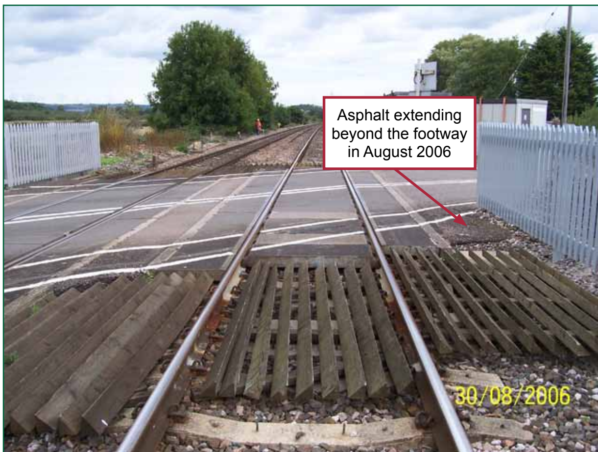
Figure 9: The asphalt section in August 2006 (photograph courtesy of Network Rail)
